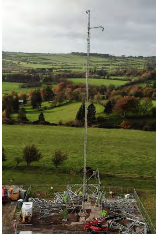
Figure 6-4 – Gin pole erected
