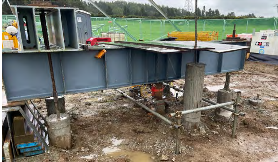
Figure 6-9 – Pile testing
