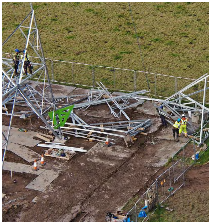
Figure 6-5 – Preparation of tower section for lifting
