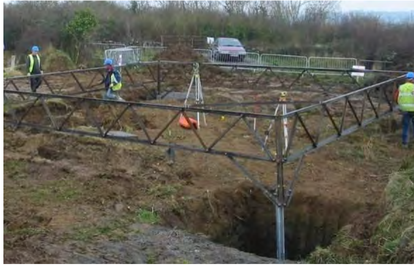
Figure 4-2 – Traditional ESB stub setting template
