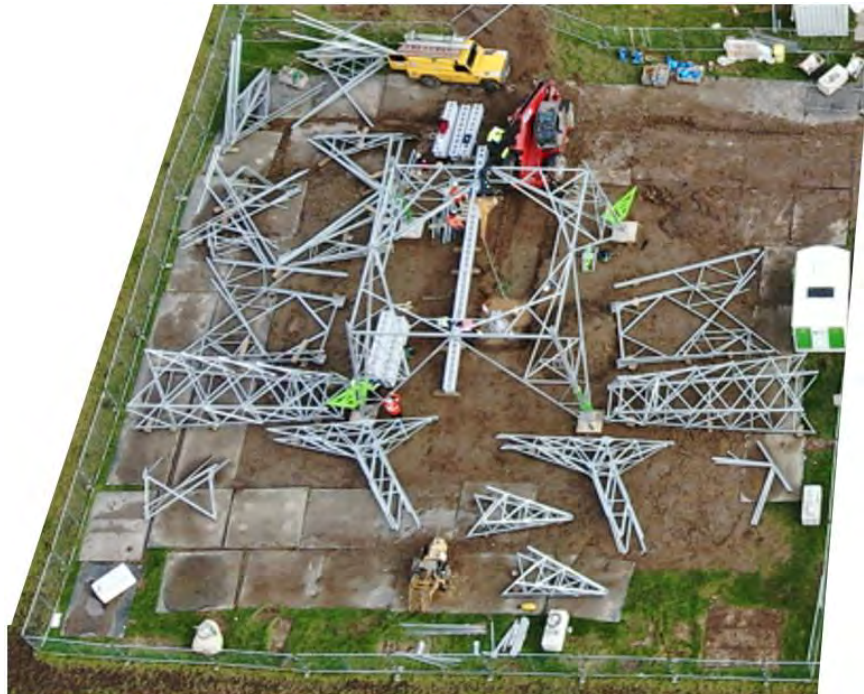
Figure 6-3 – Preassembled tower sections with tower base and second concrete pour complete
