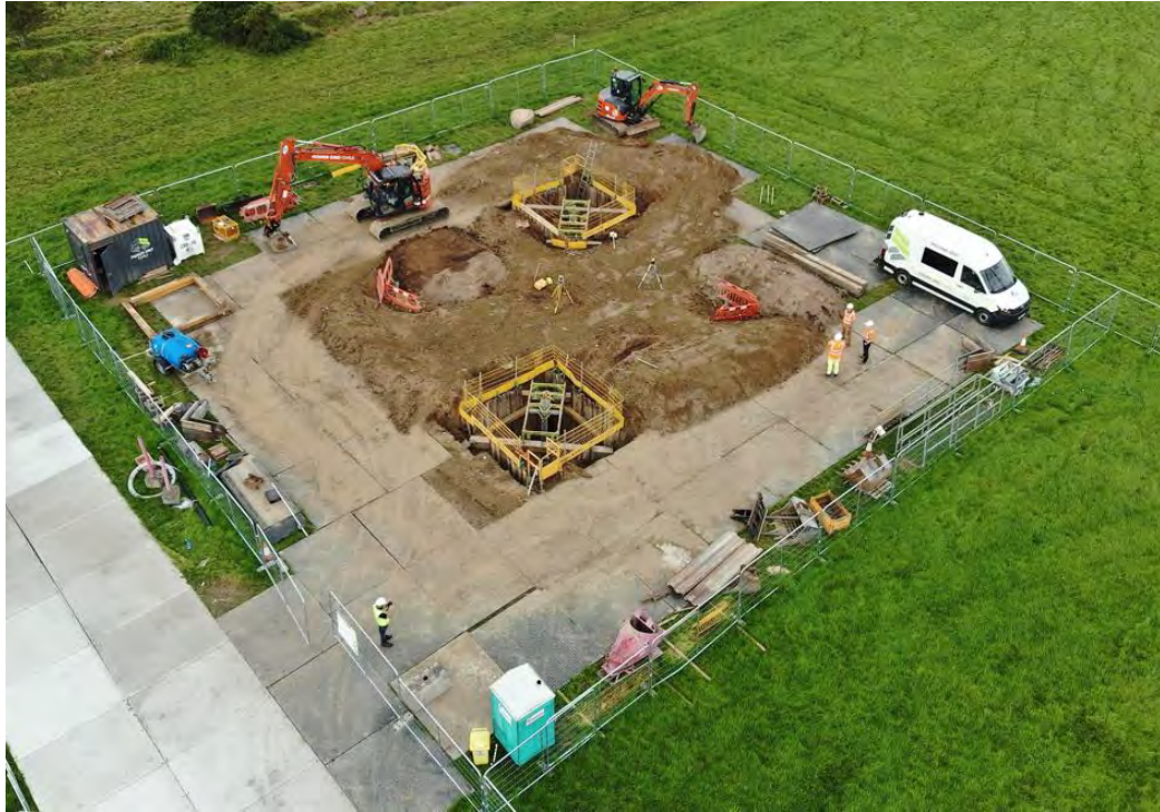
Figure 6-1 – Pad & chimney foundation stage: Works at legs 2 and 4
