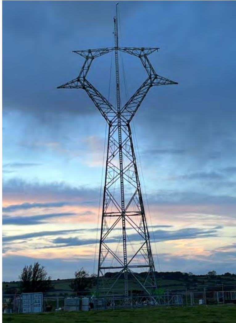
Figure 6-6 – Completed tower prior to gin pole removal
