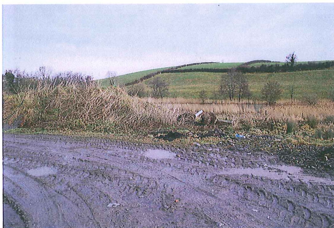
Area of recent infilling for road works.
