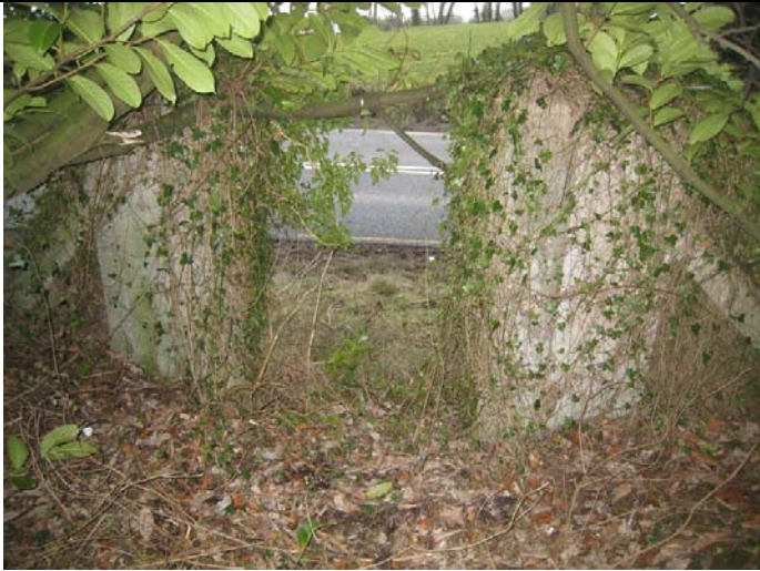
Gate from Church looking W
