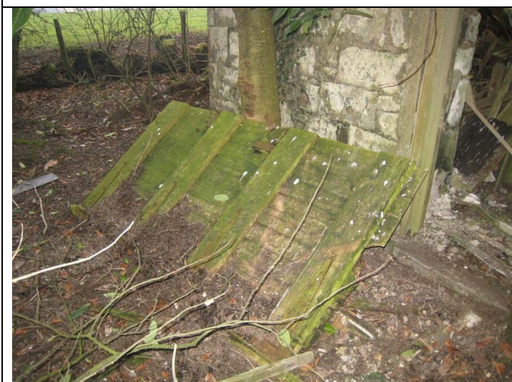
Detail of main door, door stone sill and masonry
