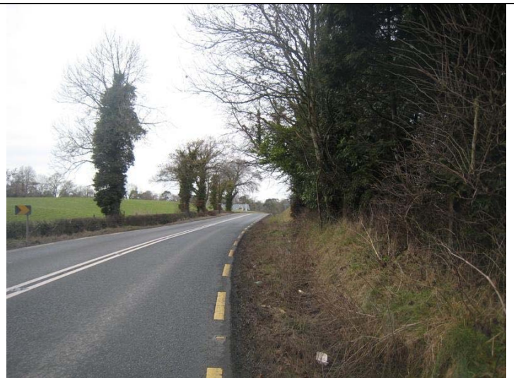
Widened N2 looking N (Church on right)
