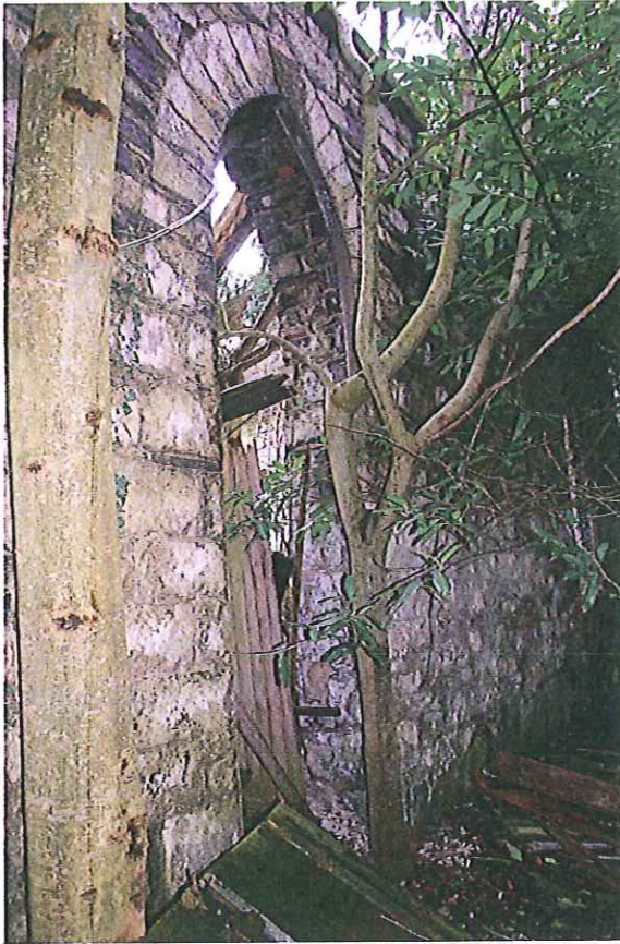
Front elevation, with main door detail.
