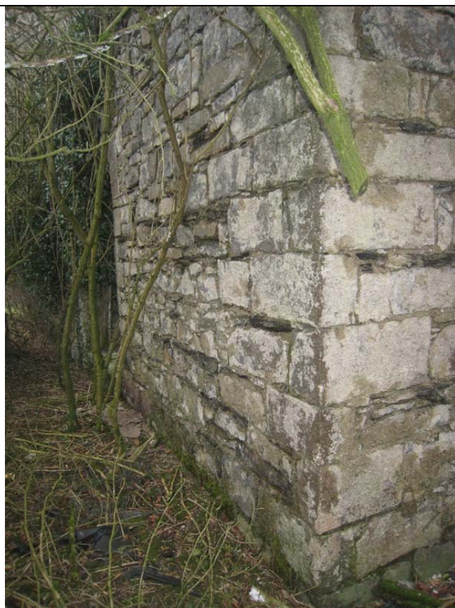
Detail of masonry on NE corner looking S along E wall
