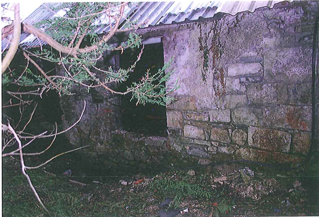
Side view, northern elevation.
