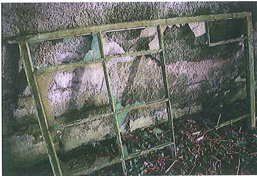
Section of timber window with coloured glass panels from gable wall.
