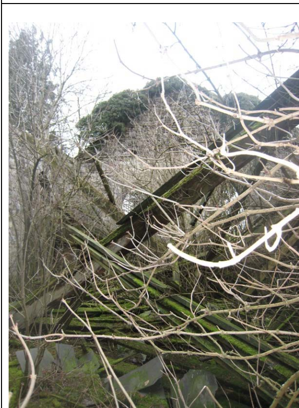
Interior from S
