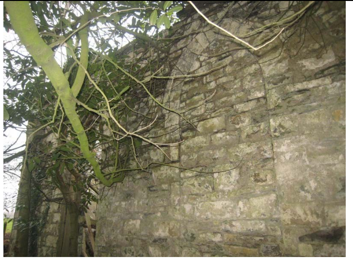
Central blocked window on W side
