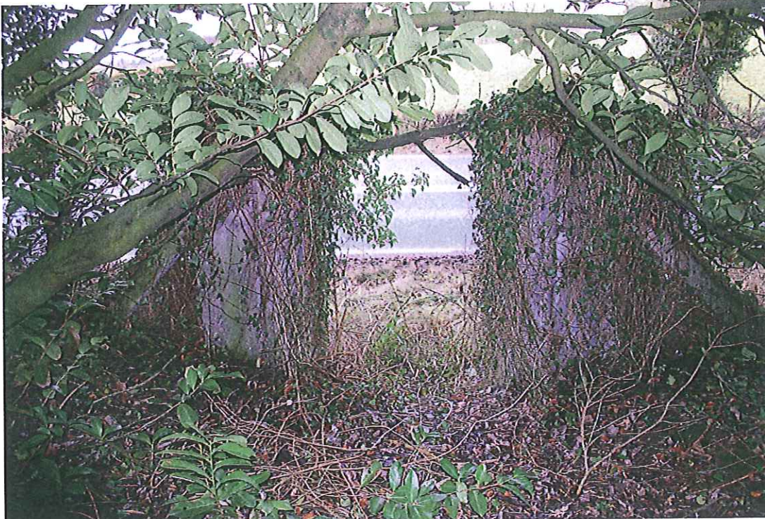
Stone entrance pillars at entrance onto N2.
