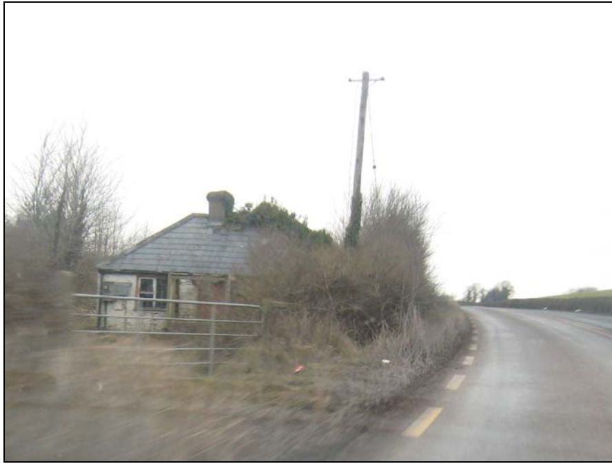
Photo of building at Ch1775. This building will require a survey if it is due to be demolished.
