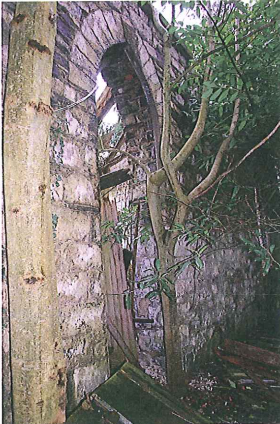
Front elevation, with main door detail.
