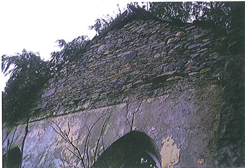
Interior gable wall.
