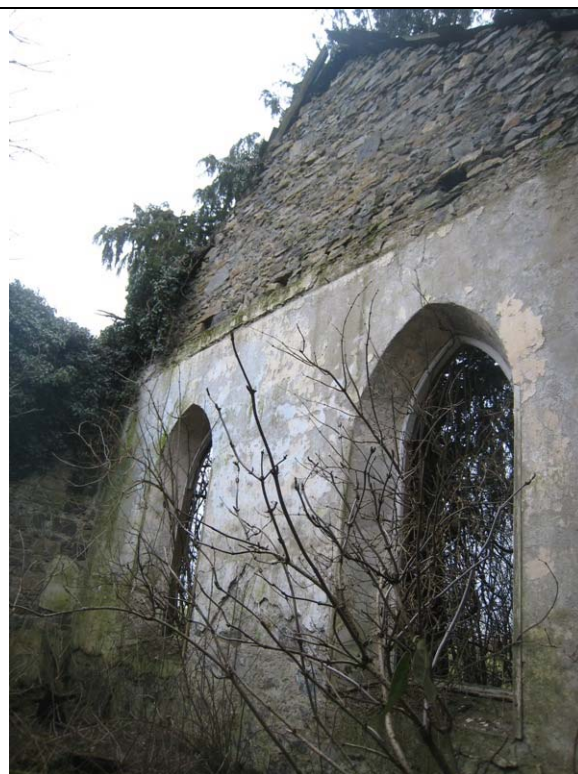
Interior of S gable wall
