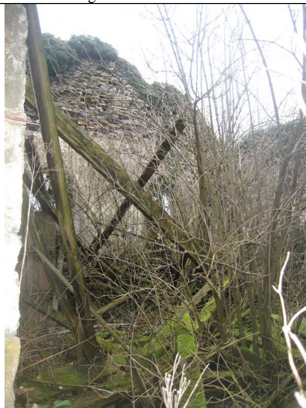
Interior N gable wall
