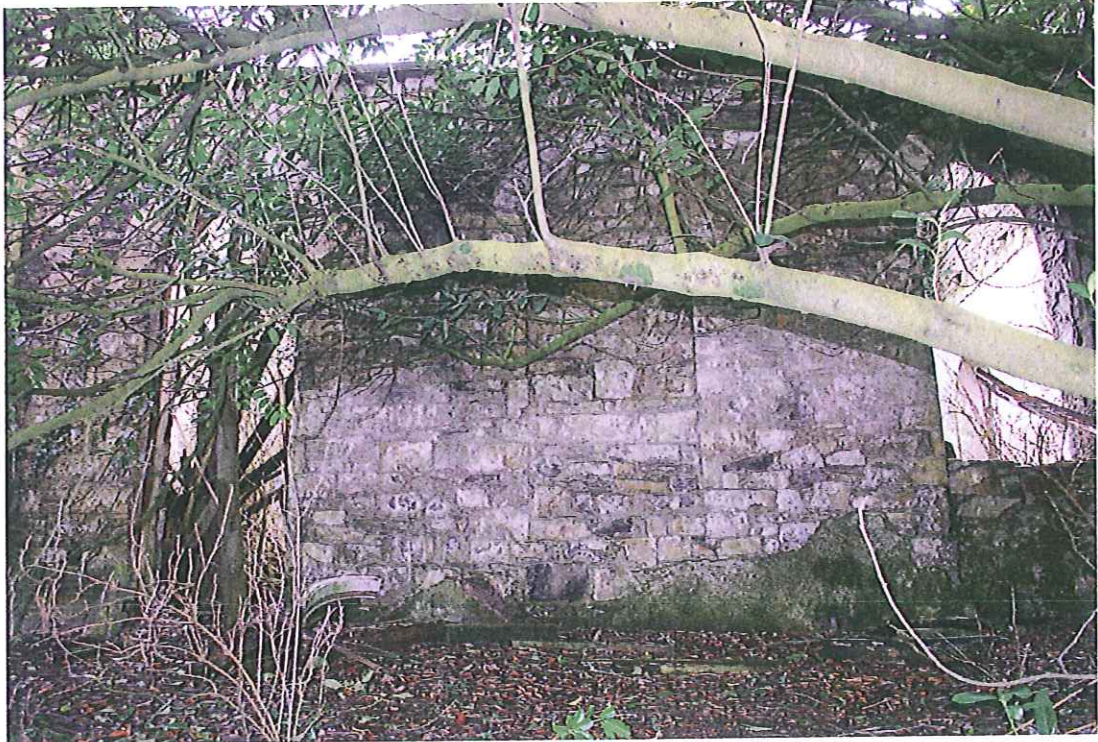
Front elevation, door to left, window to right, blocked up central window,
