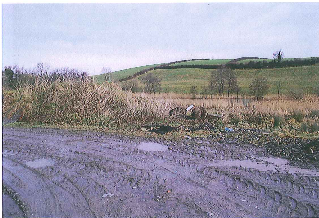
Area of recent infilling for road works.
