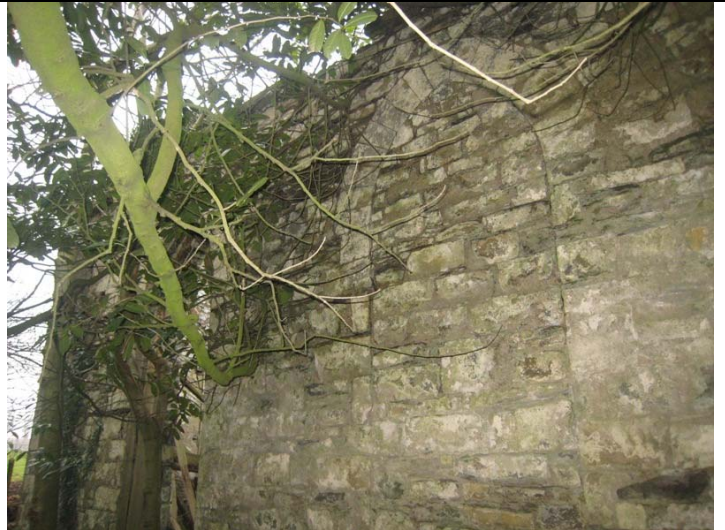
Central blocked window on W side
