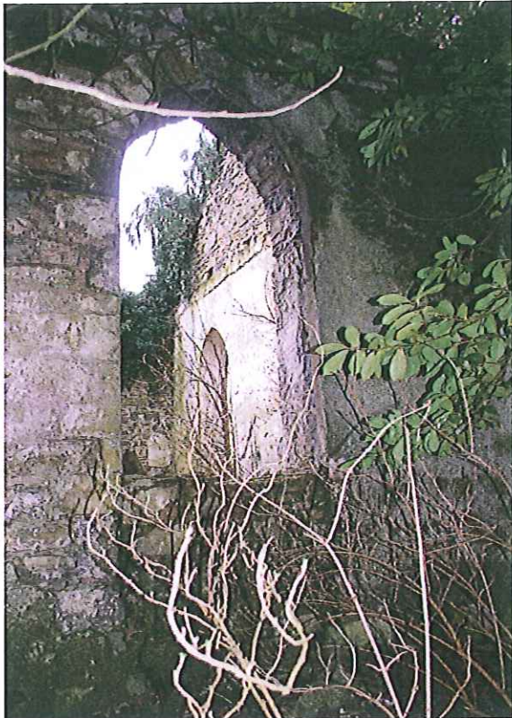
West elevation, front of church.
