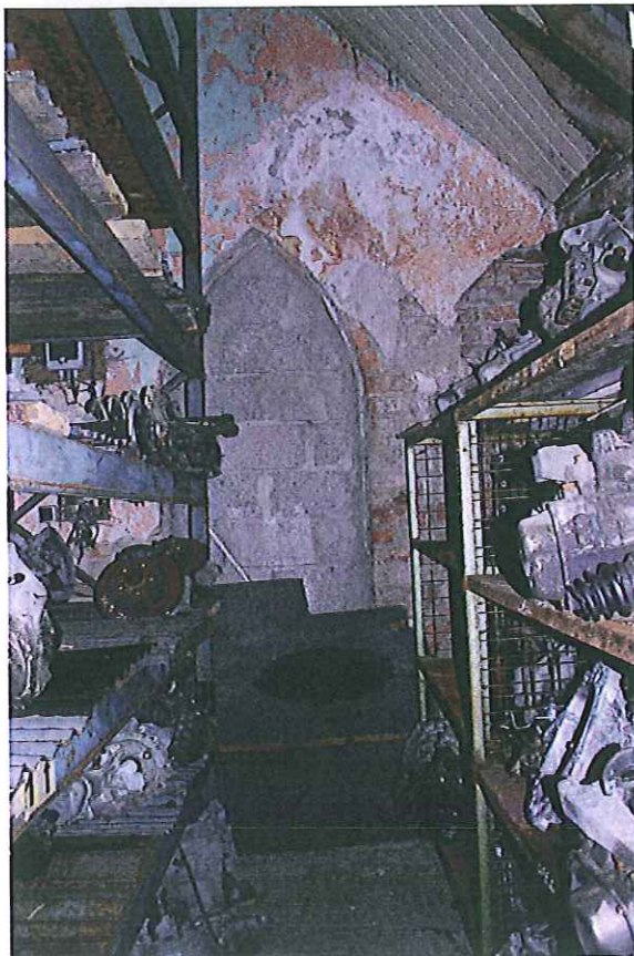
Interior, front elevation, pointed arch openings.
