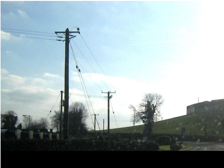
Fig 3.19: Area of Chainage 1.800 – 1.900 from the north.
