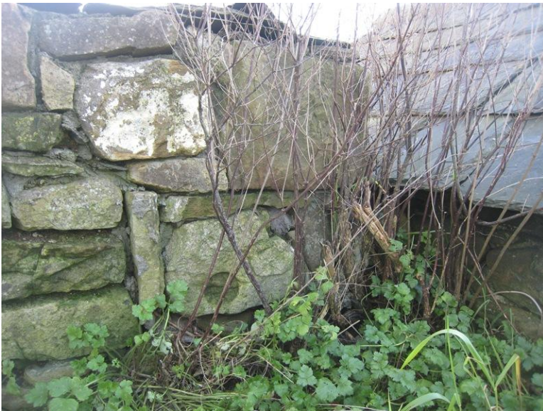
Fig 3.11: reused stone in wall between two buildings
