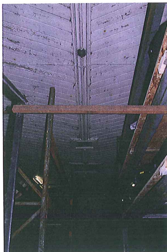
Timber battened ceiling to interior with vent detail.
