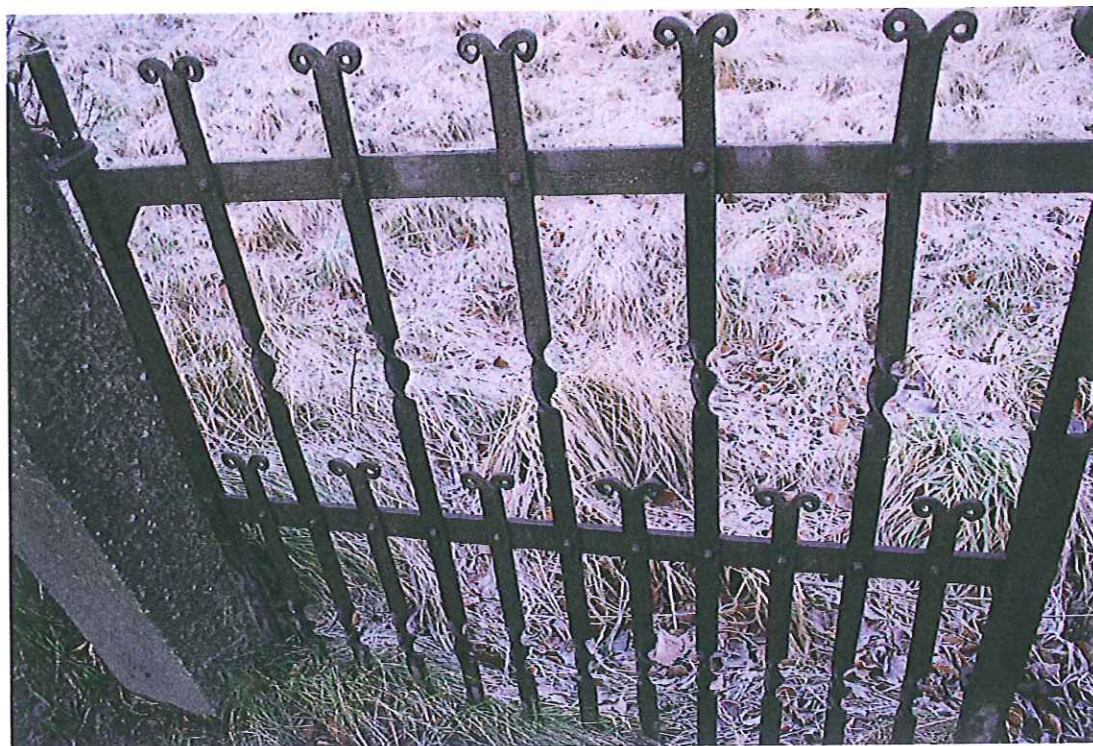
Original forged iron gates and stone pillars to meeting house site.
