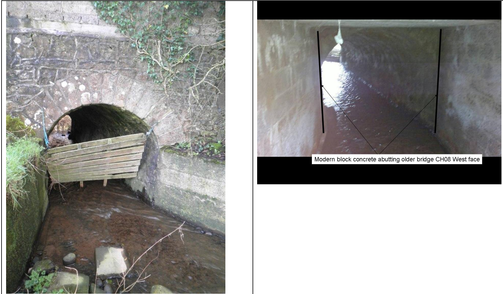
Fig 3.15b: CH08 Hoof Bridge Photographs. Left: Eastern face with concrete additions. Right: Western face with concrete additions
