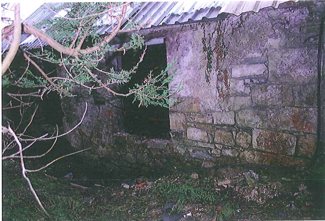
Side view, northern elevation.
