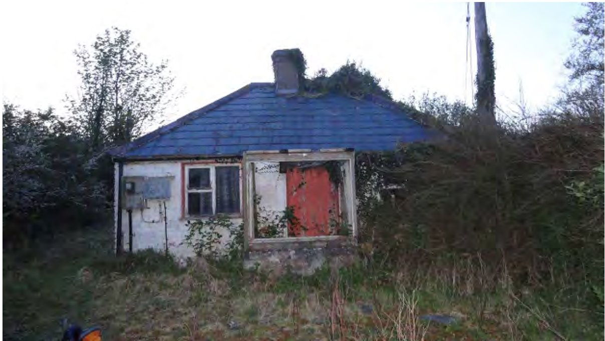
Plate 1: Cottage (Site 1) located along the N2 existing road (west of route).
