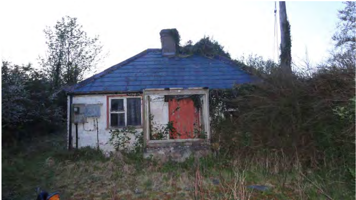
Plate 1: Cottage (Site 1) located along the N2 existing road (west of route).
