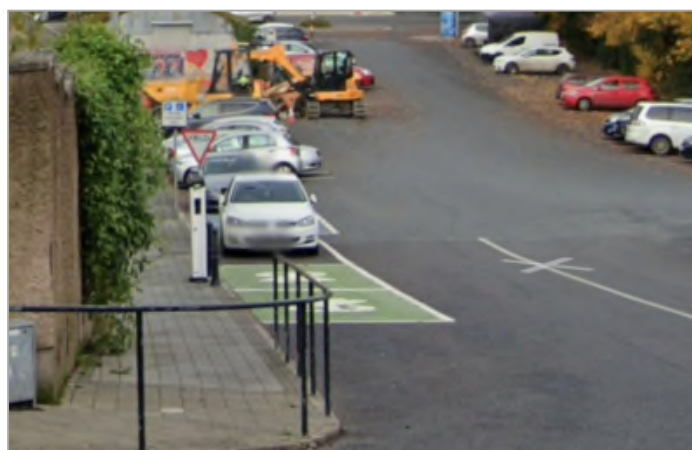
Figure 3-35 EV charging point at Town Centre Car Park
