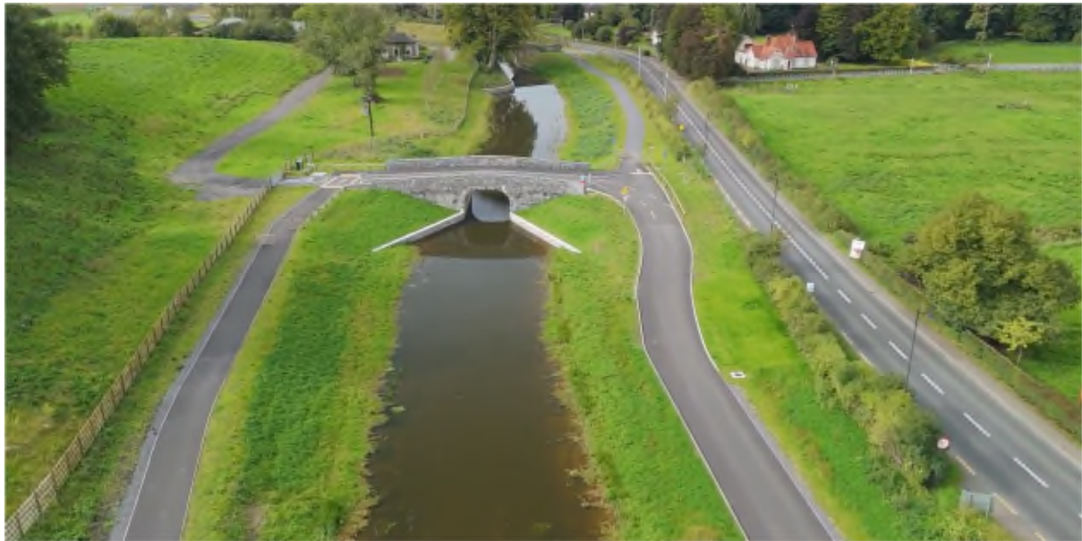
Figure 3-28 Existing active travel infrastructure south of the Marina parallel to the N54
