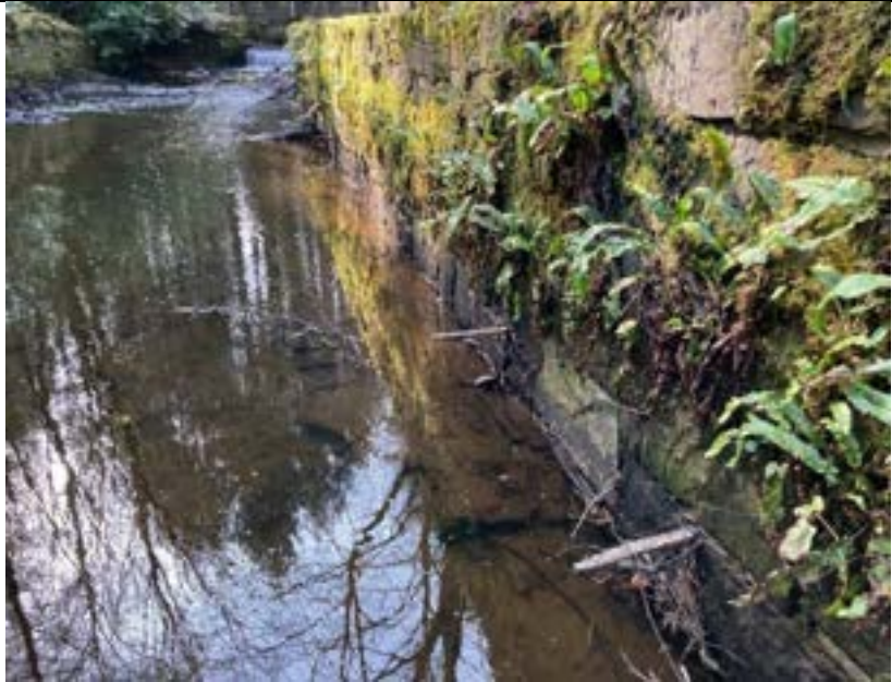
Iron brackets for piping
