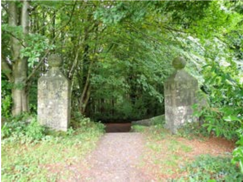
Leaning piers, especially the pier on the right of the image
