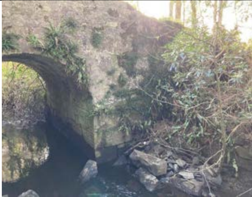
Parapet stones rest by the stream. Tree growing from retaining stone wall.
