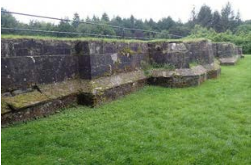
Ashlar limestone walls on chamfered plinth with inappropriate railings
