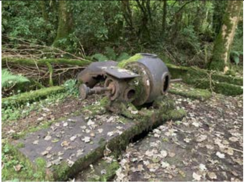
Pumping machinery in detail. Note corrosion on underside of large pipe which carried water from the tank to the south east up on the hill
