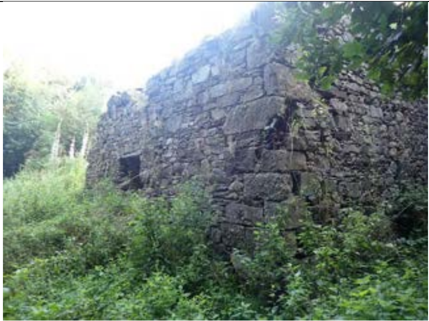
Rear exterior of Barn/Pavilion with window ope visible
