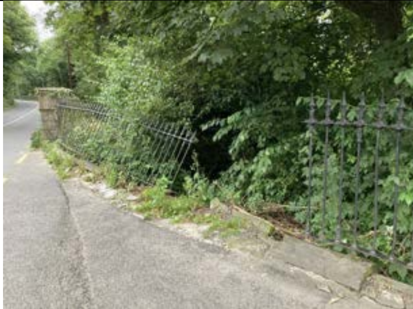
Area of collapse. Railings and plinth are still on site, albeit damaged.
