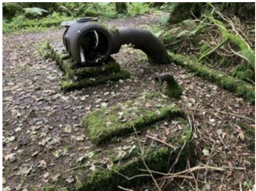
Pumping machinery in detail
