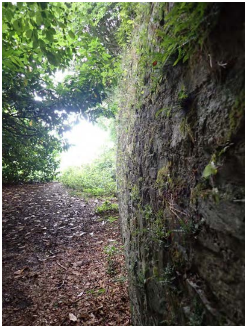
Bulge in the screen wall
