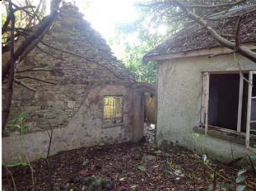
Exterior of cottage with outbuilding to left. Note carved limestone arch.
