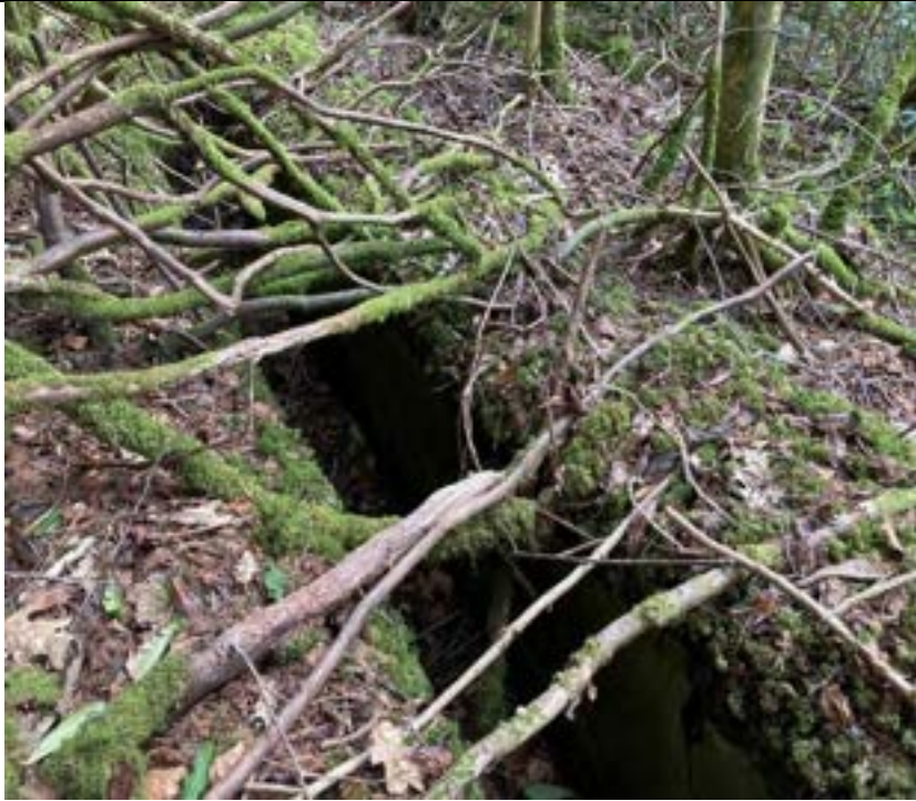
Inside the mill race are rendered walls
