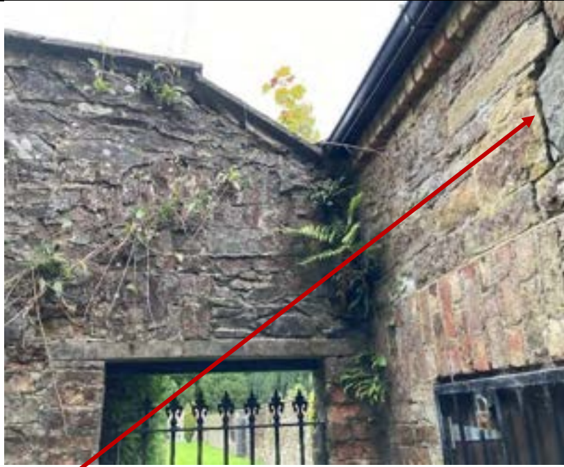
Large crack visible on two storey, pitched roof structure. Concrete pointing and capping also visible on the garden wall.
