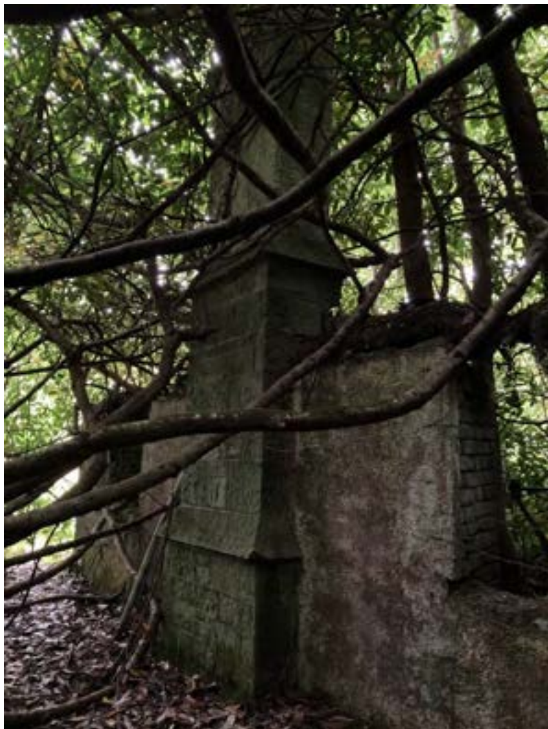
One of the two standing limestone chimney stacks
