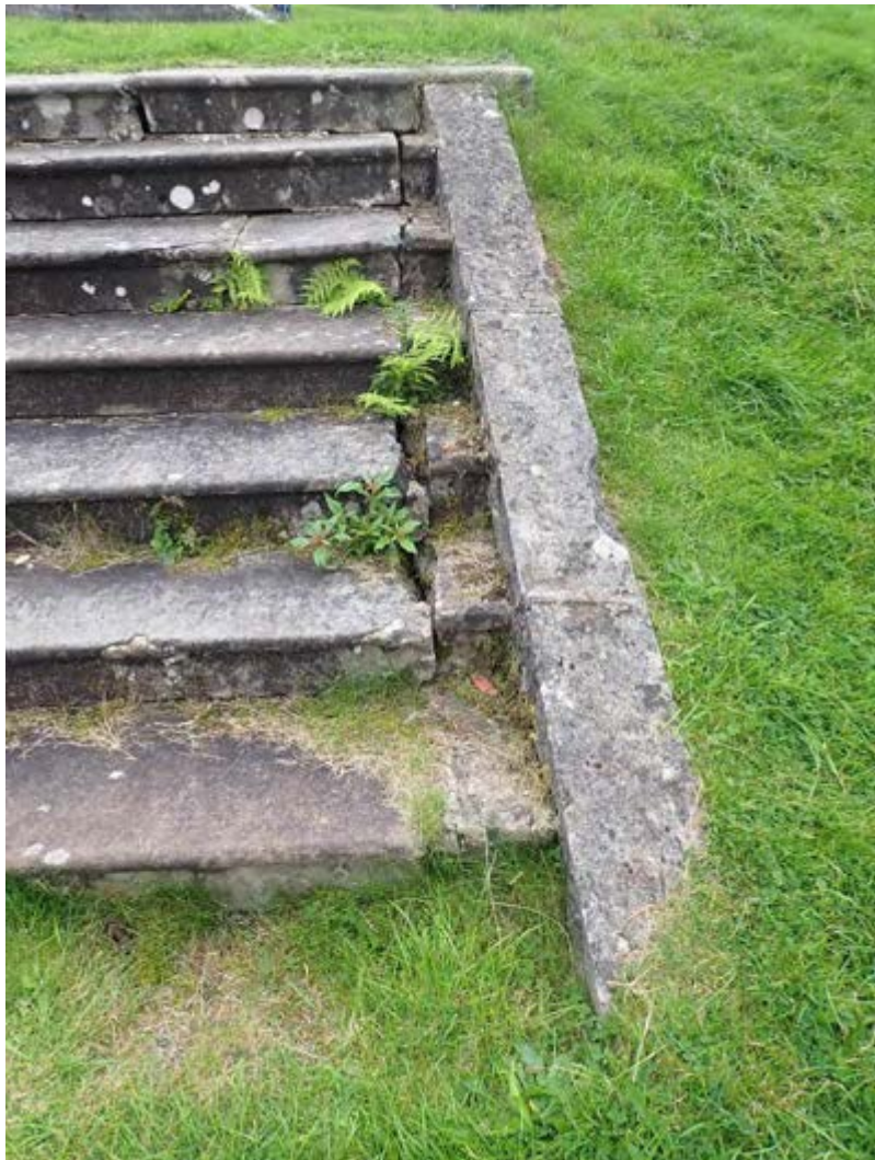
Uneven top step, gaps between stones, concrete repairs and vegetation growth are all visible
