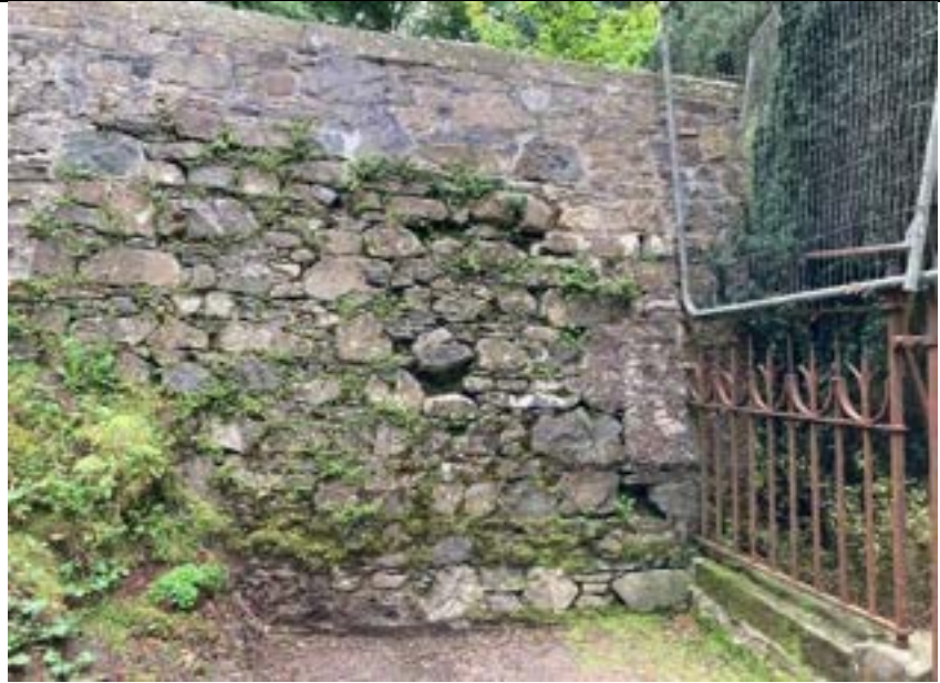
Graveyard wall with missing stones
