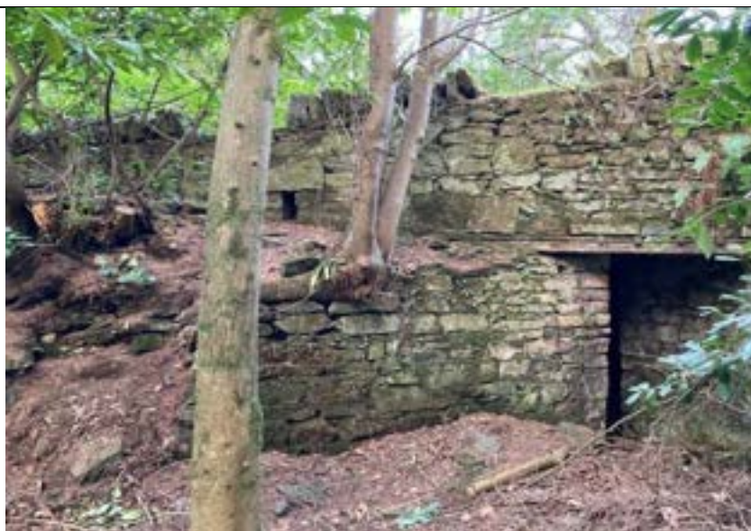
Entrance to passageway with large tree growing from reveal wall head
