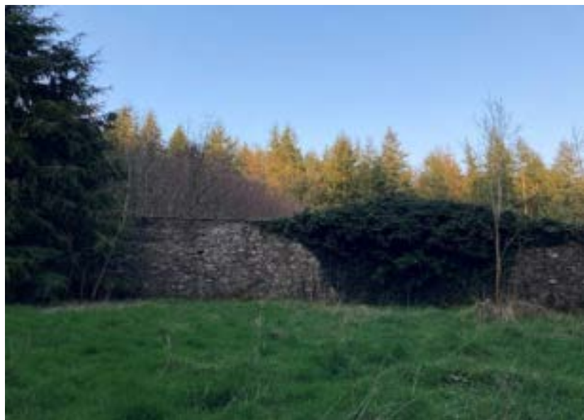
Enclosure wall with missing stones, missing pointing and stretches of extensive ivy growth
