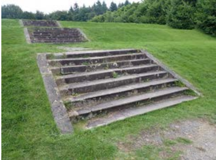
Three of the five sets of steps. Note worn grass in foreground
