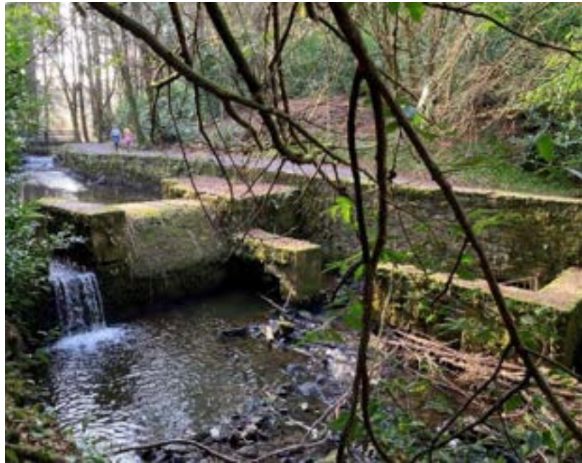
View of dam and area for ram taken from mill race
