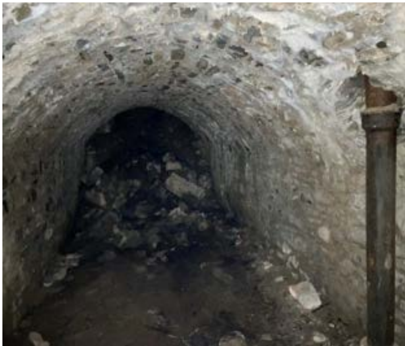
Interior of passageway with pipe associated with outside tank
