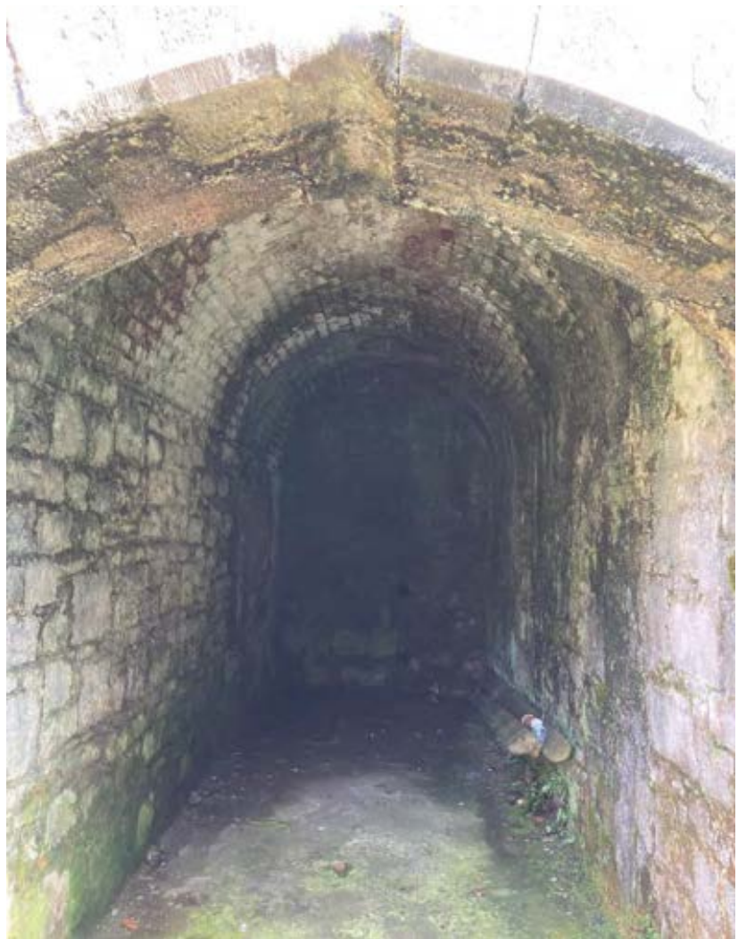
Interior of Servant's Entrance. Passageway blocked.
