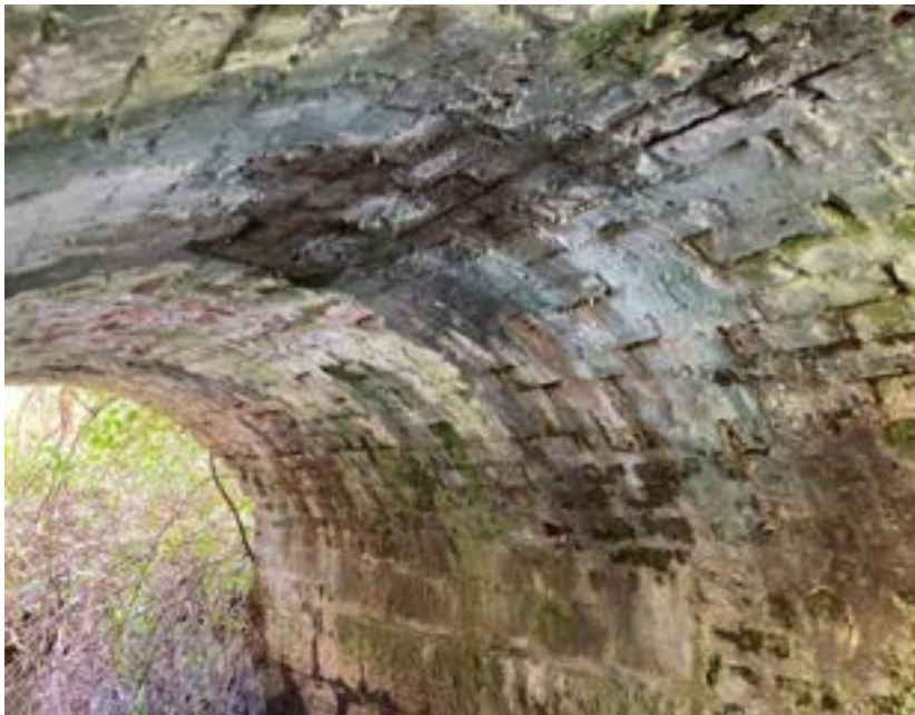
Brick underside of arch
