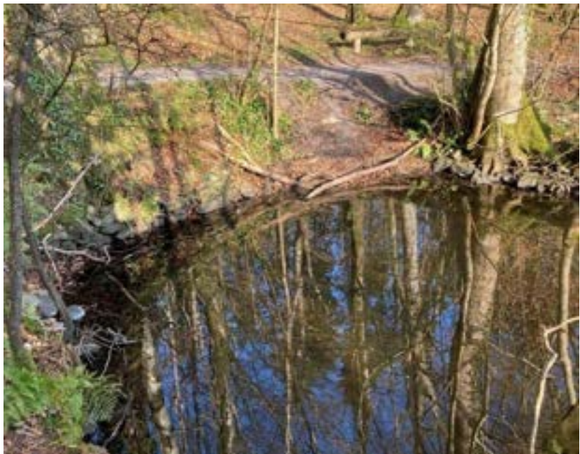
View of boathouse stone foundations/footings.
