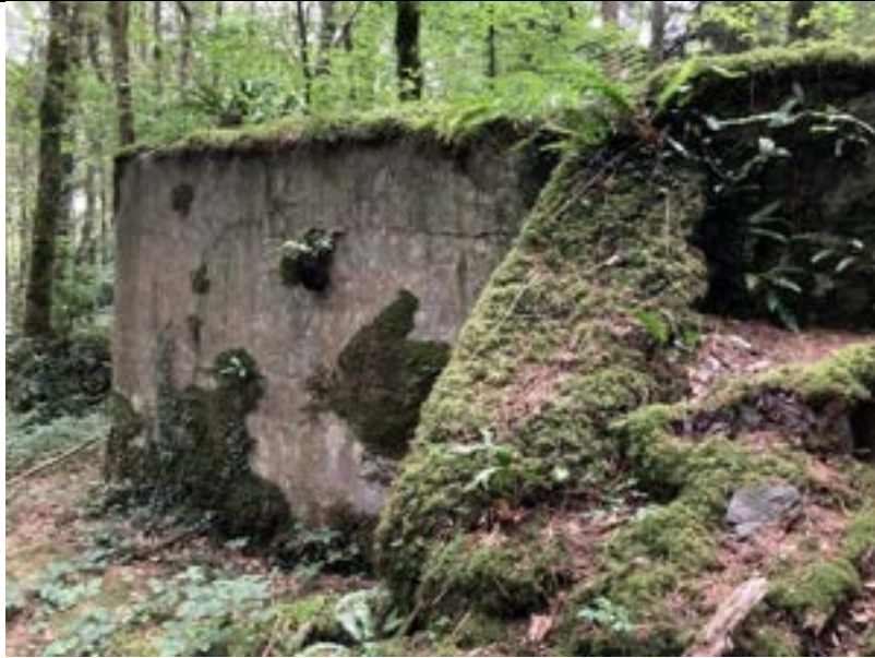
Rendered walls with cracking and vegetation growth
