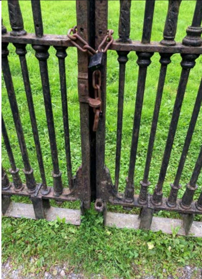
The gates are missing various decorative elements. The latch is also partially missing. Later steel additions have been added at the base.
