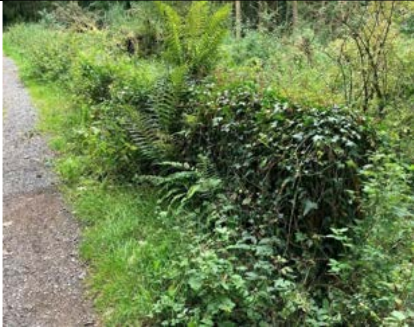
Southern parapet wall is covered in vegetation
