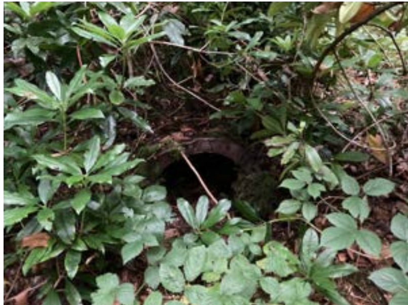
Probable wrought iron piping leading from the tank to the Engine House. This piping is not indicated on the Historic 25" OS map.
