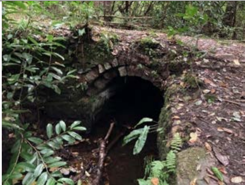
East side of bridge. No handrail present.
