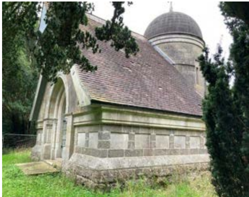
Missing slates in the roof
