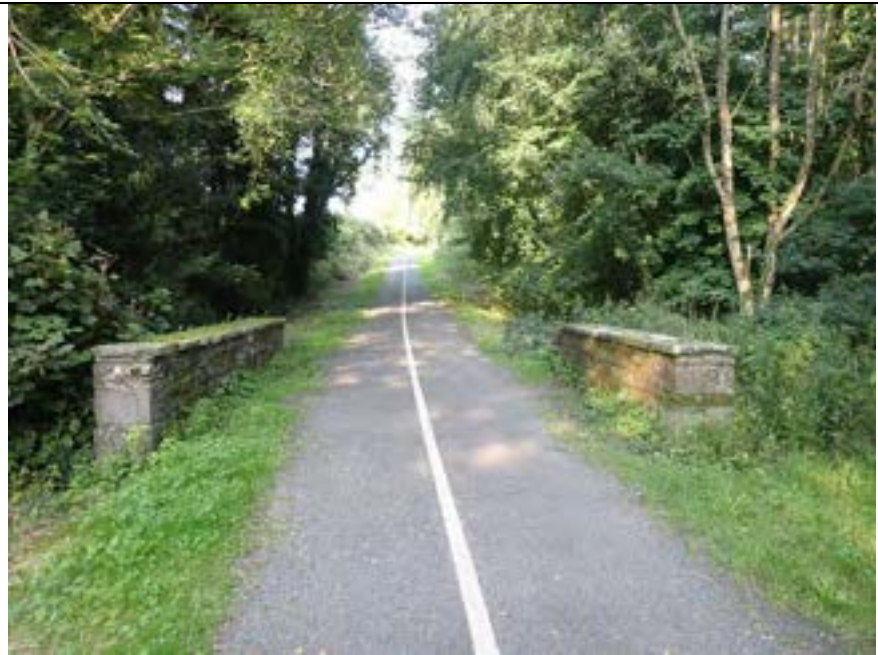
Bridge looking northeast
