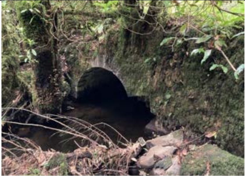
Missing stones in arch and heavy vegetation growth is obvious
