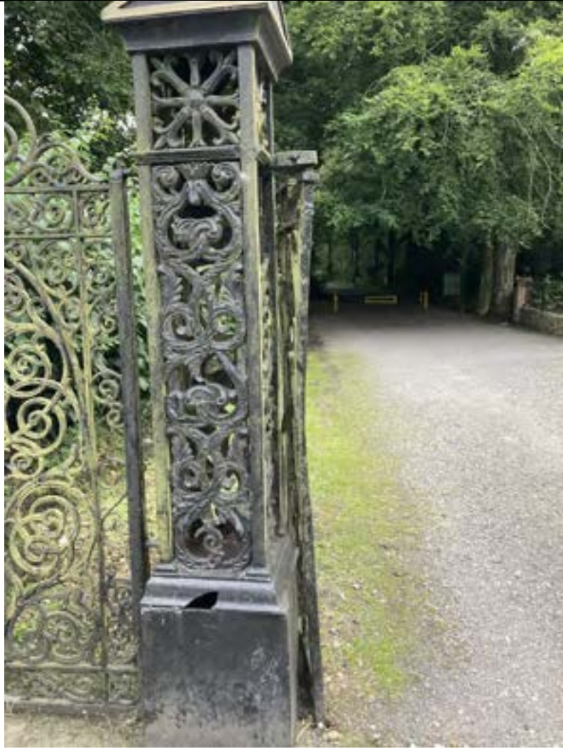
Broken piece allowing water and debris into the structure. There is a noticeable bend in the gate. Was this caused by Mick Jagger?
