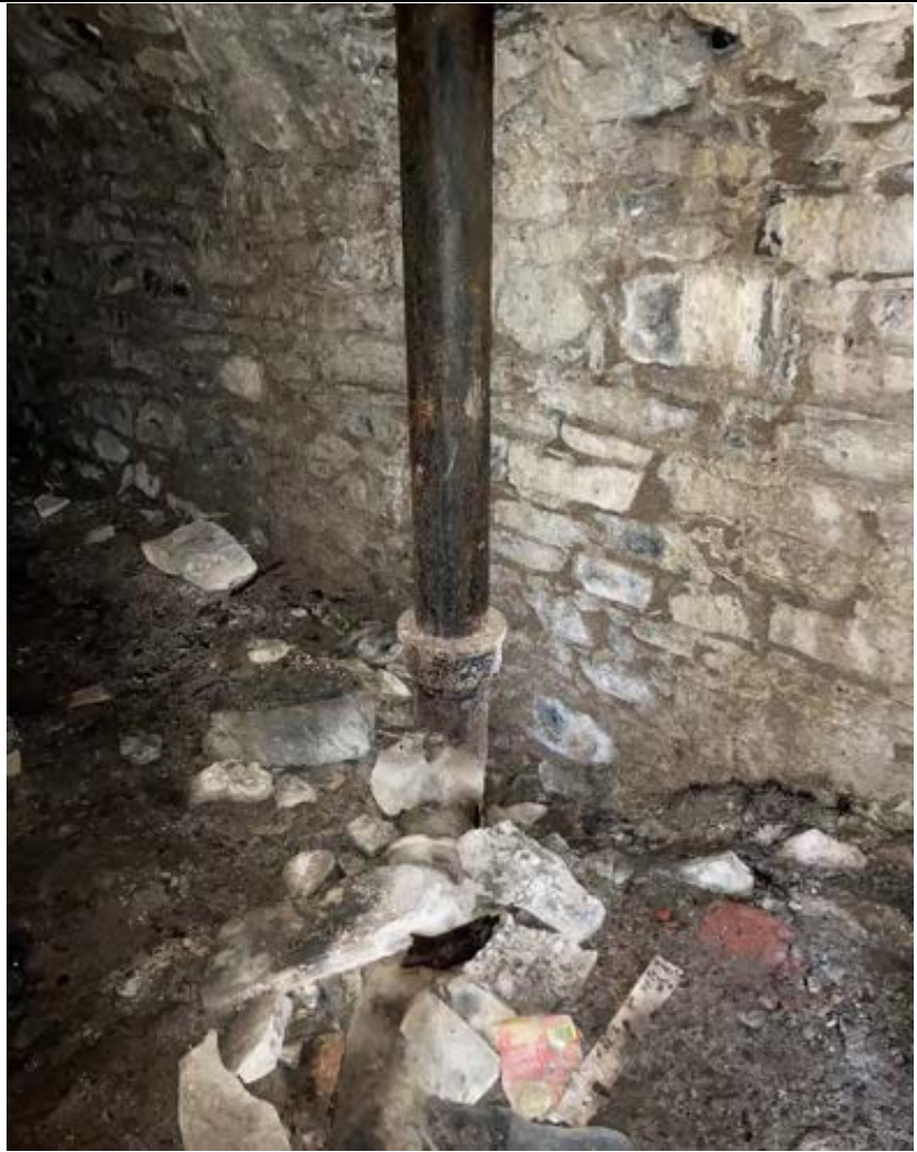
Iron water pipe (wastewater?) in adjacent underground passage which leads to the tank
