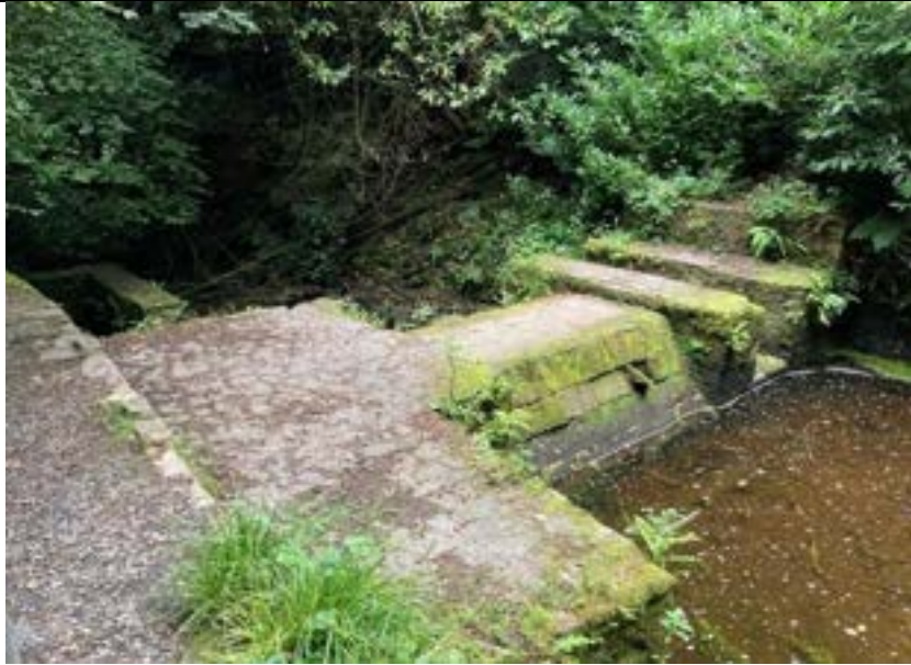
Dam with dislodged ashlar stones
