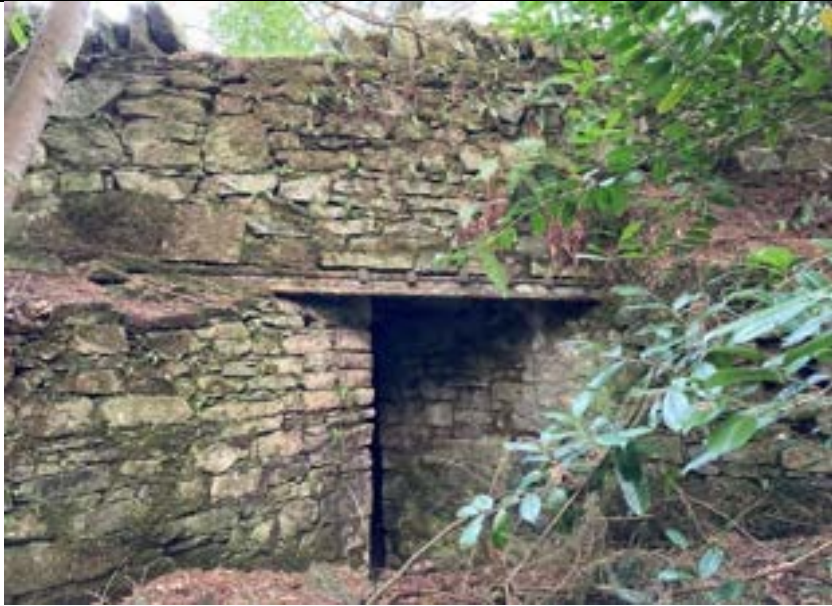
Entrance to passageway with main routeway from carpark to castle above
