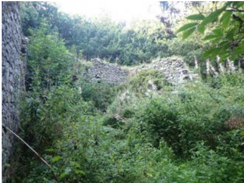
Interior of structure
