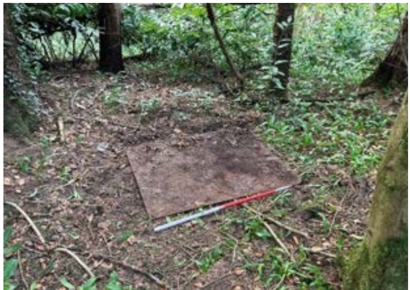
Loose steel plate over the hatch. Image taken looking from nearby passageway entrance
