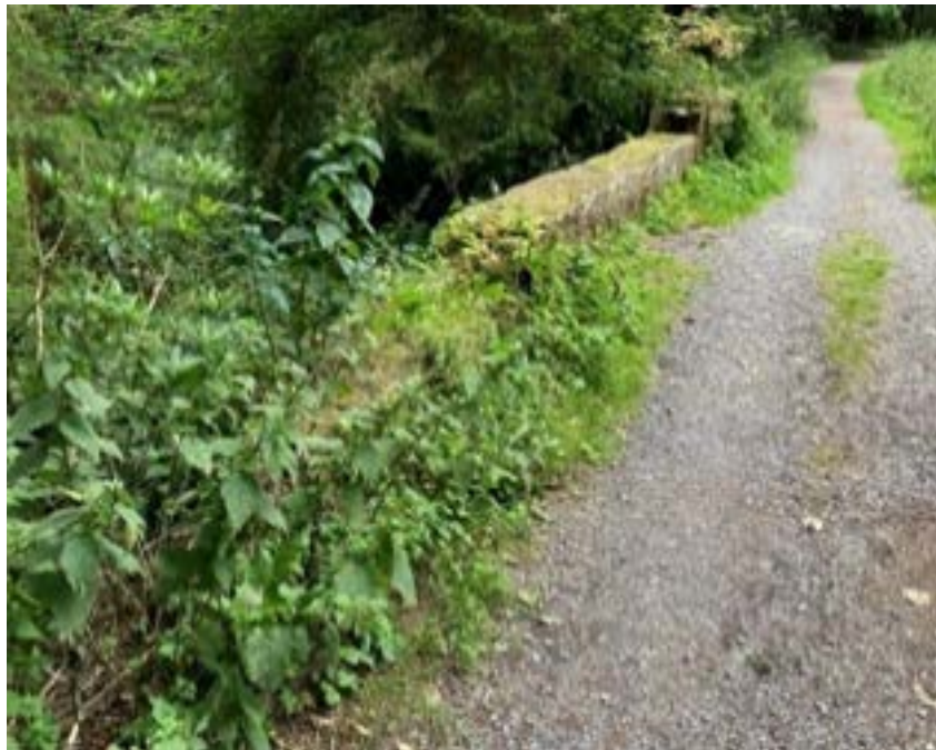
Much of the north parapet has been demolished
