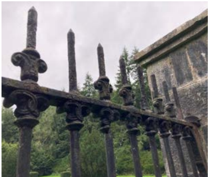
Some of the broken and missing elements of the gate
