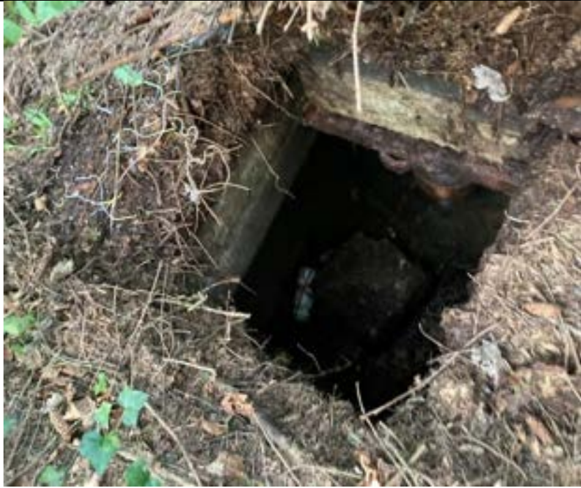
Hatch with tank underneath
