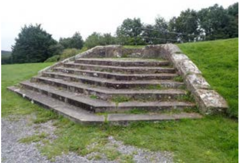
Corner steps, now uneven
