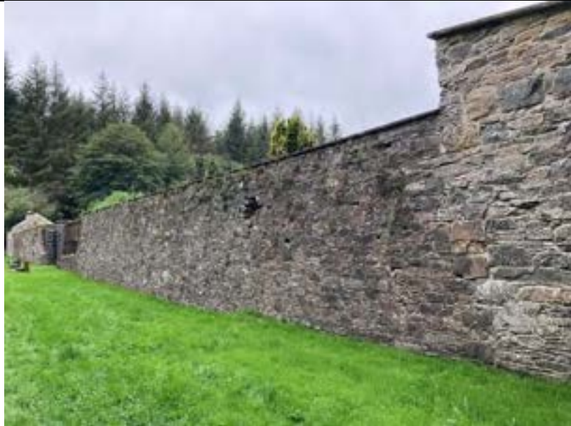
Southeast wall with main entrance. Several missing stones in the wall are visible.
