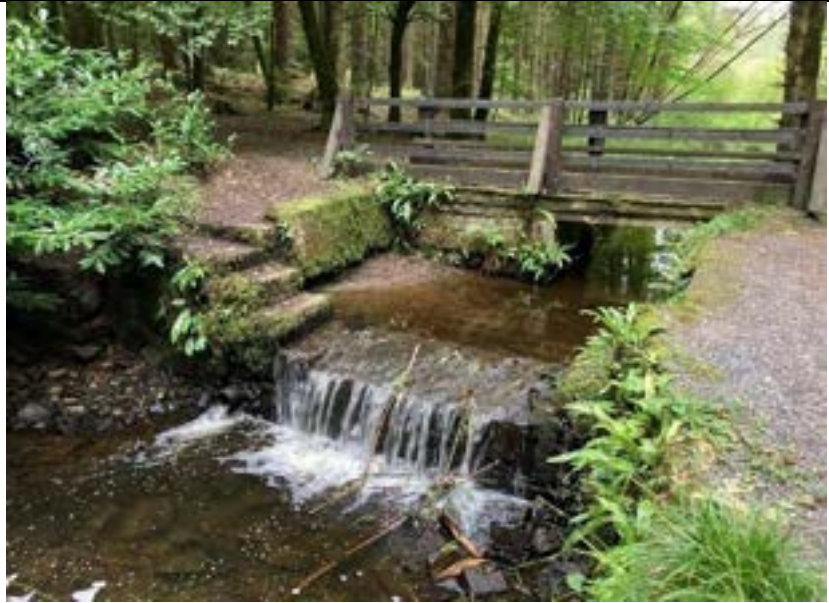
Weir just upstream from the dam. Vegetation growth and water erosion visible on retaining walls
