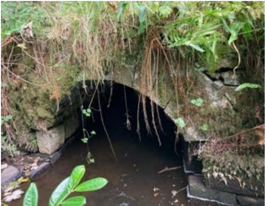
Missing and loose stones in arch. Failed pointing in spandrels.
