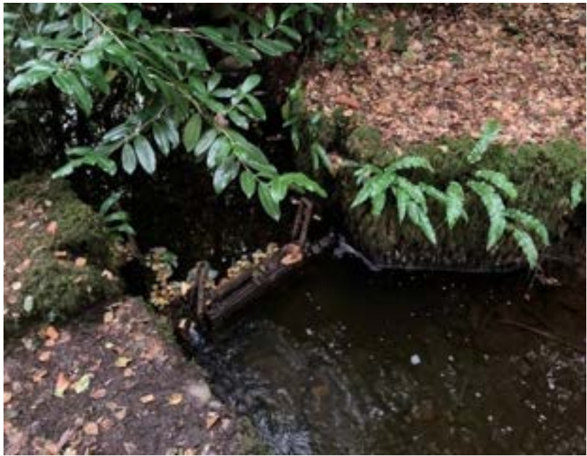
Cast iron sluice gate
