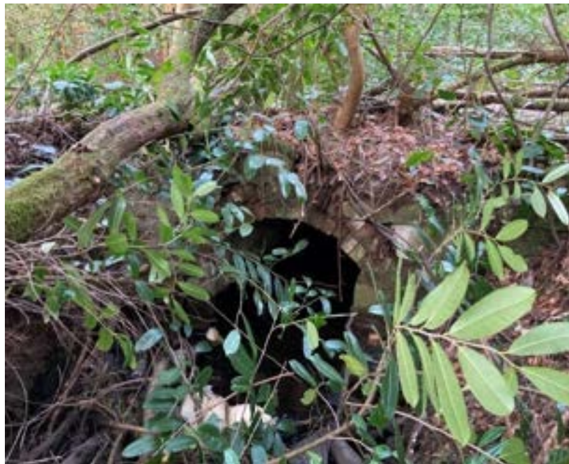
West side of bridge
