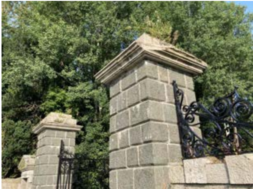
Vegetation growth on top of piers. Damaged stonework also visible.
