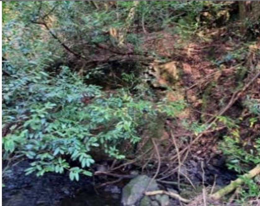
The beginnings of the mill race. Photo taken from dam. Taken from dam, beginning of mill race. Section missing that connected with stream.
