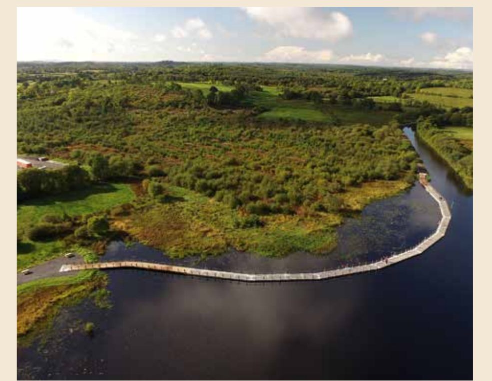
Flood Resistant Boardwalk, Acres, Co. Leitrim
