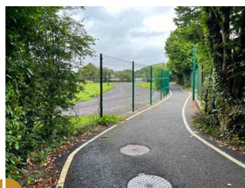
Fenced Canal Greenway Sections
