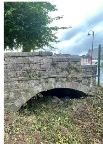
Ulster Canal Bridge, Old Cross Square
