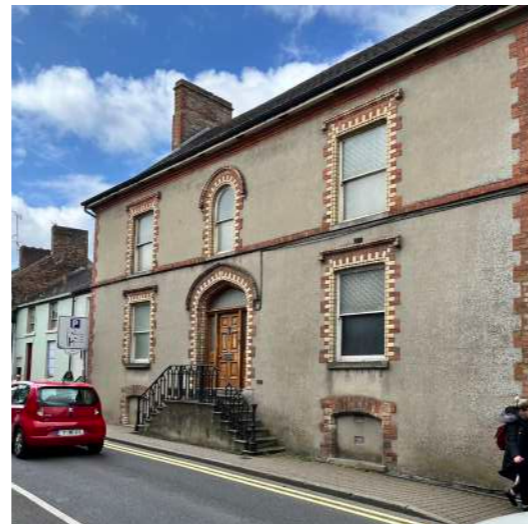
14. Young Memorial Masonic Hall, 37 Glaslough Street, 1880
