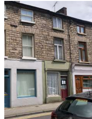
Wool Shop, 47 Dublin Street
