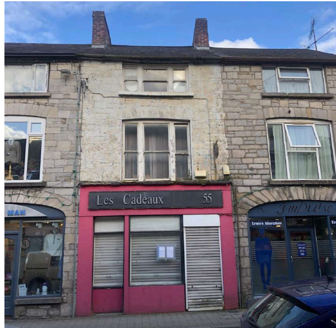
Current view of no. 54,55 and 56 Dublin Street
