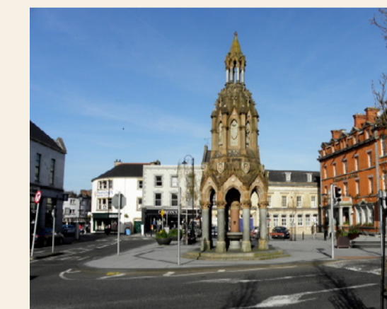
H10 Rossmore Monument Restoration
