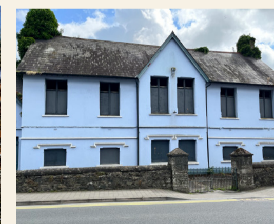
H13 Assembly Rooms Façade Restoration and Pocket Parks
