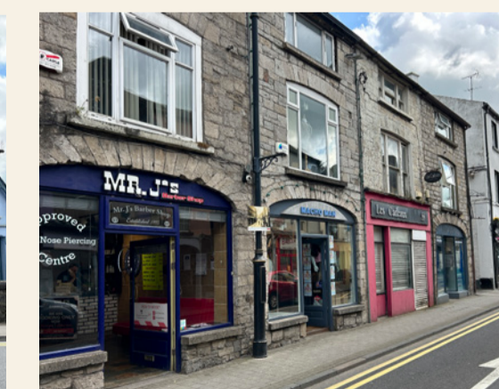
H14 No. 54-57 Dublin Street Façade Restoration
