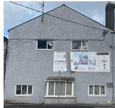
Old Civil Defence building, Monaghan Town
