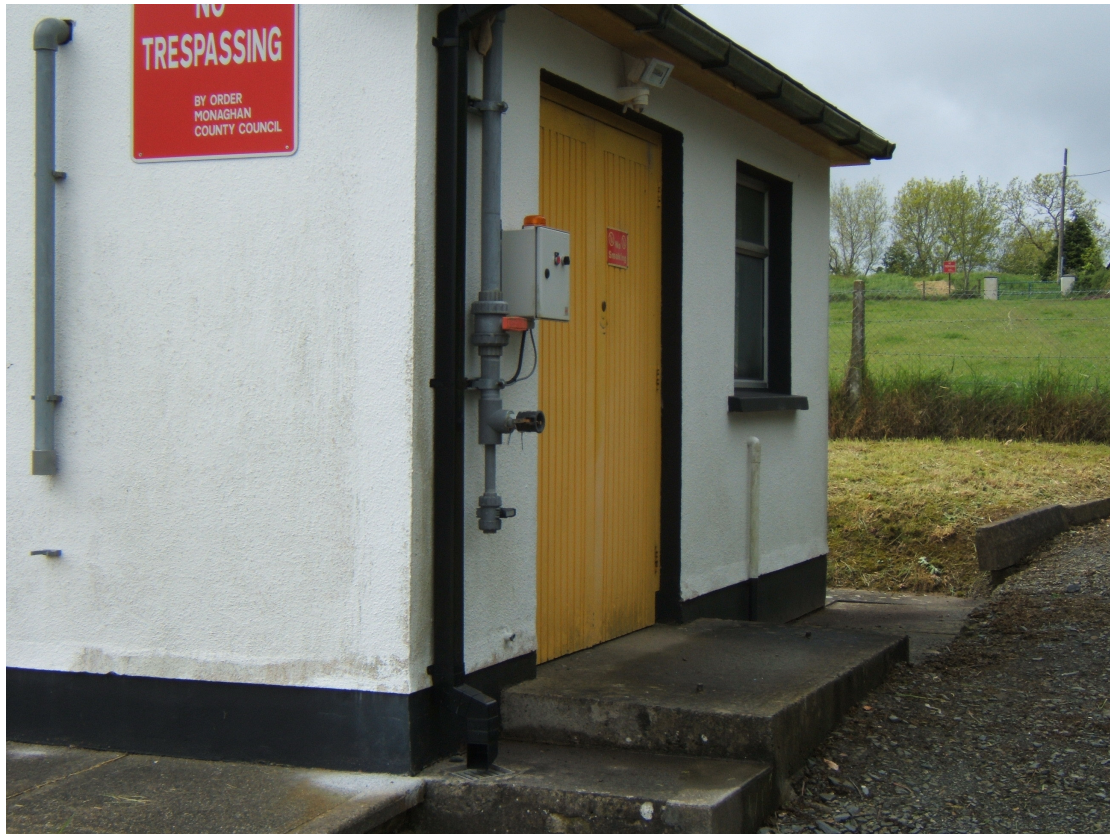
Photo 5. Fill Point for Fluoride Bulk Storage Tank.
