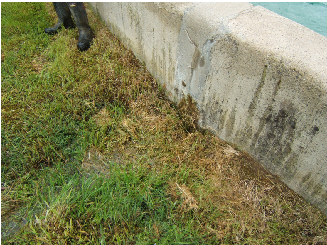
Photo 4. Crack in the Nafferty Reservoir (note outflow of water from crack).
