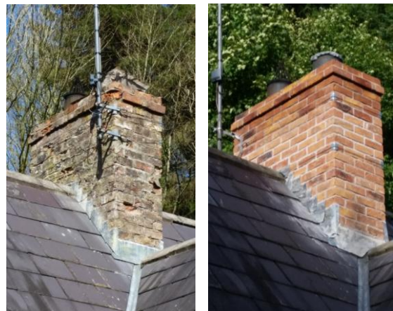
A new gate lodge chimney which addressed serious water ingress, health and safety and aesthetic issues at the Newbliss (Road Gate) Lodge, Rossmore Park, Monaghan.
