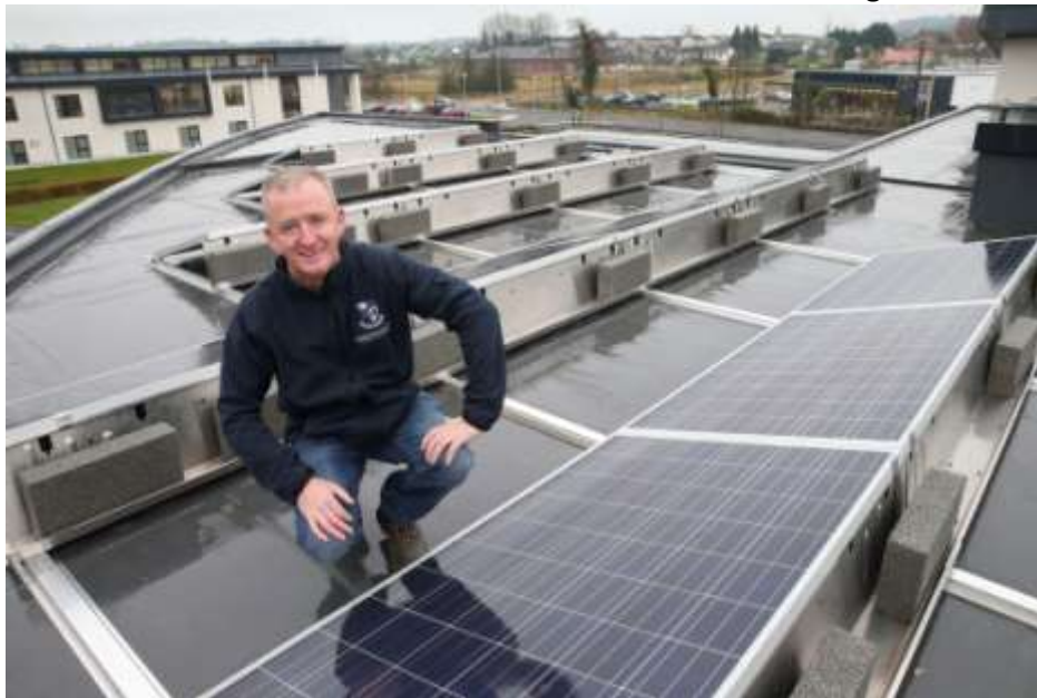
New PV Solar Panels at Carrickmacross Civic Building
