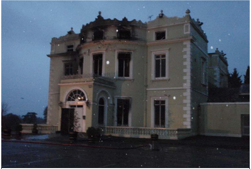
Fire damaged Hope Castle
