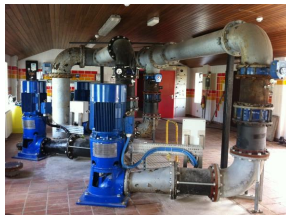
New raw water pumps at Corlea
