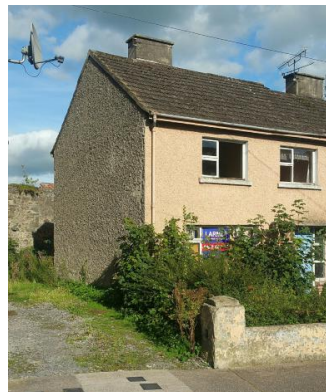
1 Analore Street, Clones: Before
