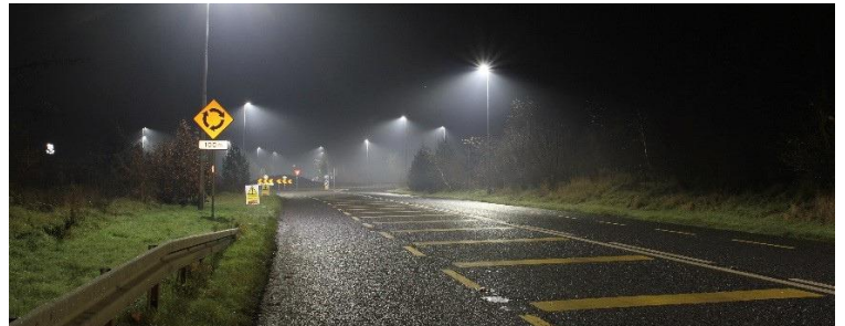
New LED lighting at Annahagh Roundabout, Monaghan Town bypass
