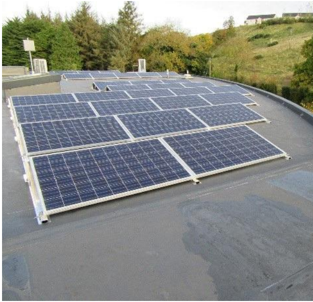
PV panel installation on roof of CMX Civic Offices
