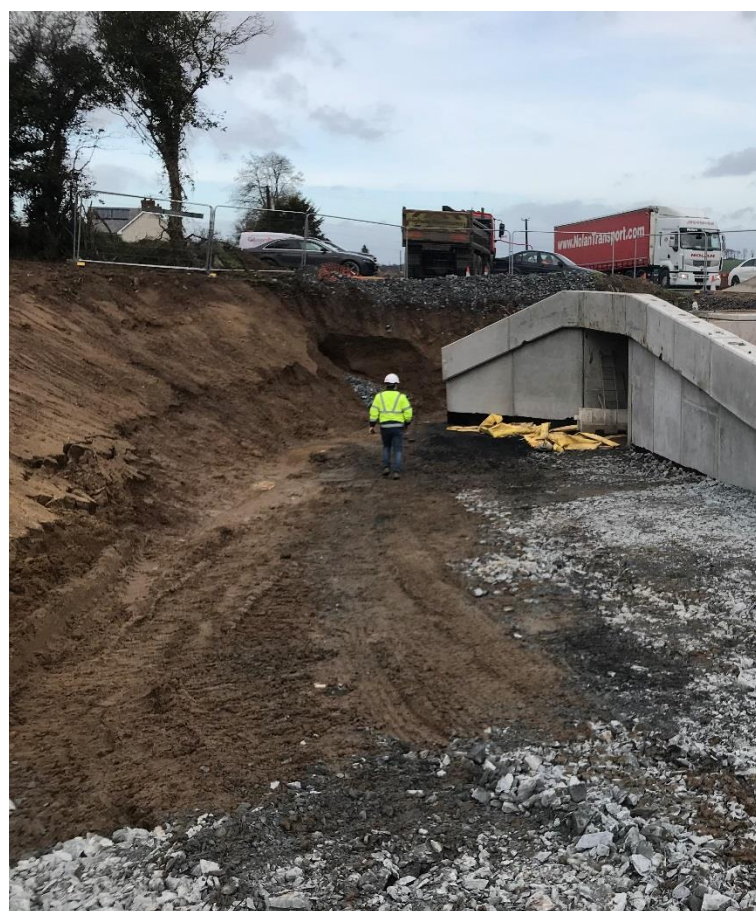
Underpass being constructed on the N2 Phase 3 realignment.
