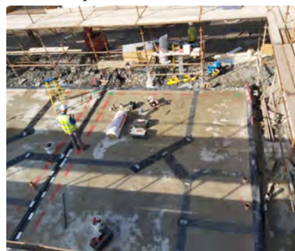
Photo above: Floor plan to line up module being lifted into place - September 2020
