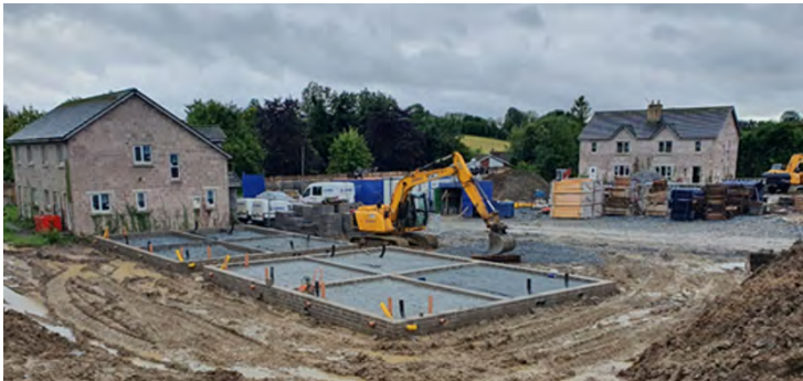
Site 2 - Former Boyle Sports site
