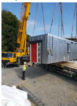
Photos above: Module being lifted into place - September 2020
