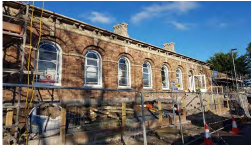
Windows at the Station Master's House, Kilnacloy (Built Heritage Investment Scheme)
