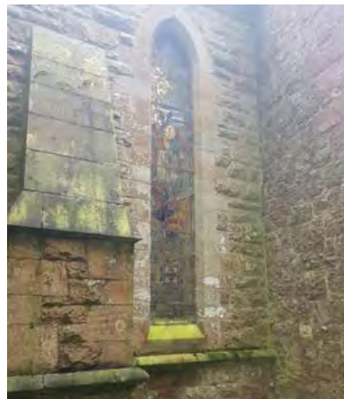
Stained glass window repairs and storm glazing at St Salvator's Glaslough (Built Heritage Investment Scheme)
