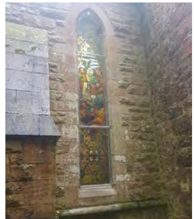
Stained glass window repairs and storm glazing at St Salvator's Glaslough (Built Heritage Investment Scheme)
