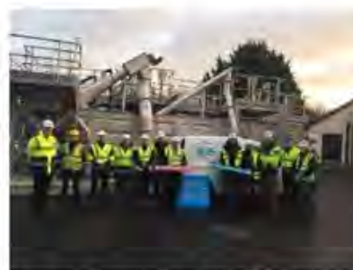
New Wastewater Treatment Plant Castleblayney – Cost €4.4m
