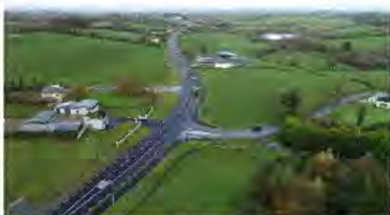
Aerial view of N2 Phase 3 Scheme.
