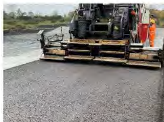
Reclaimed asphalt pilot trial.
