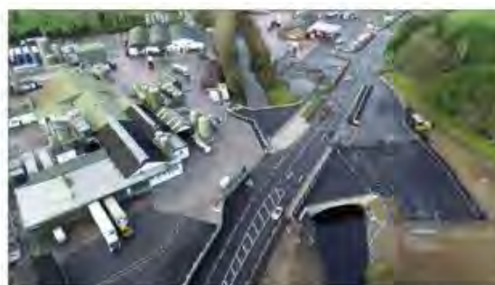
Ariel view of the Blackwater Bridge scheme and accommodation works.
