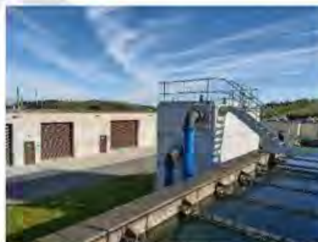
Upgrade works Kilkitt Water Treatment Plan
