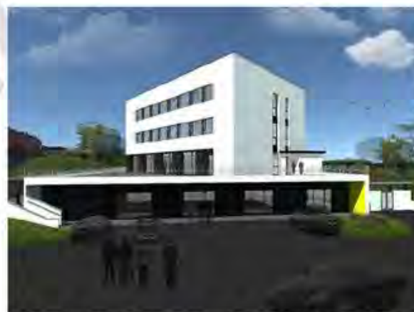
"The Ridge" Enterprise Hub, McGrath Road, Castleblayney
