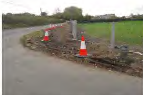
Low cost safety works, at Coolmuckbane, Monaghan MD.
