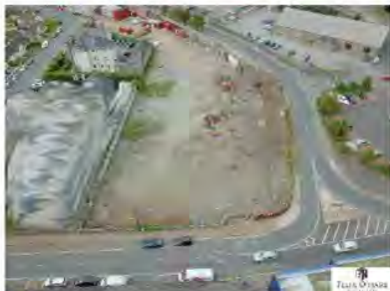
Progress in August 2020
