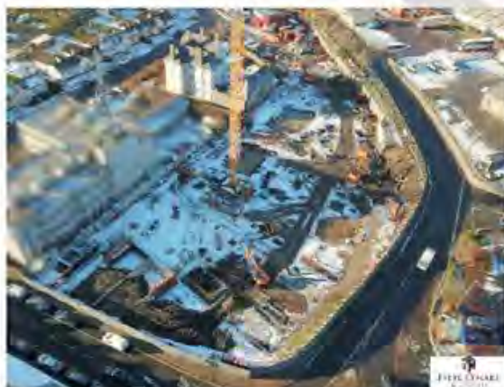
Progress in December 2020
