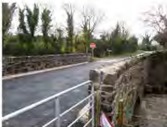
Corskea Bridge Rehabilitation works.
