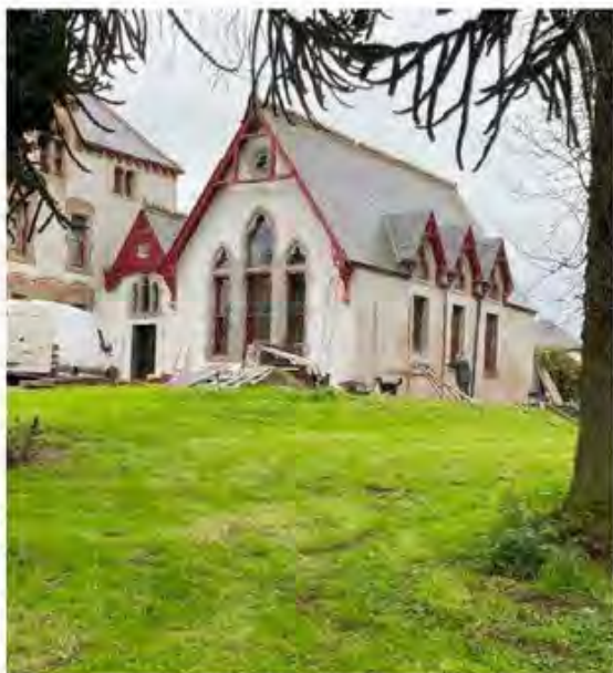
Repair of external lime render to Bessmount Park House, Music Room
