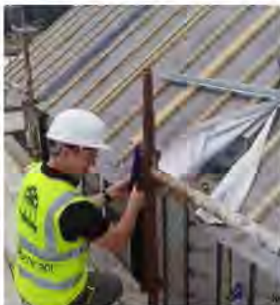
Building Control Inspection Sept 2020
