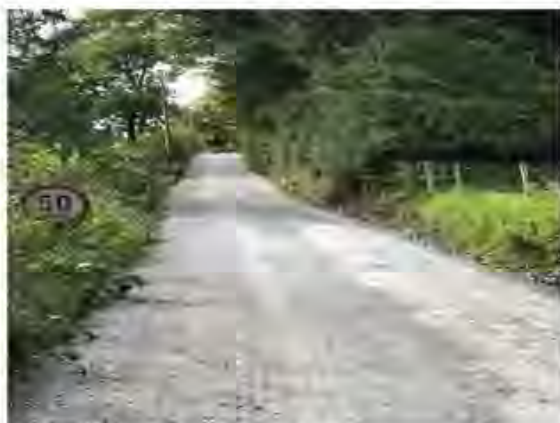
CBGM resurfacing in progress
