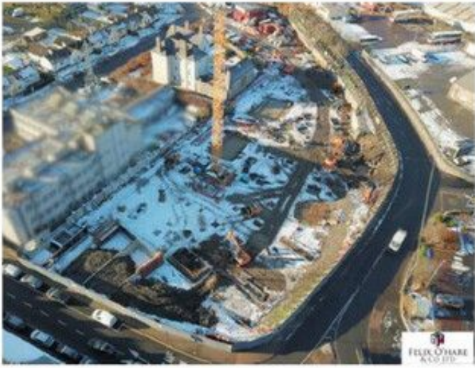
Image of site from 08/01/21 at point of Covid shutdown
