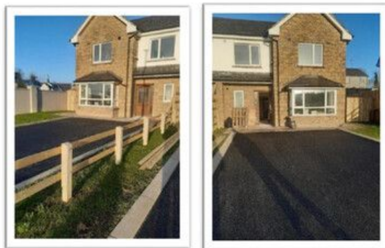
Tarmacing complete and boundary fencing erected
