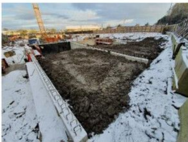
Podium ramp walls ready to pour, postponed due to cold weather.
