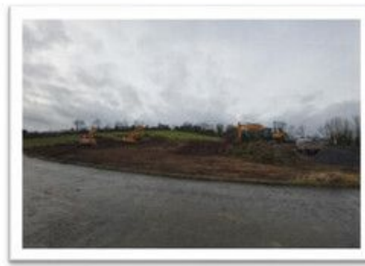
Early construction activity on site
