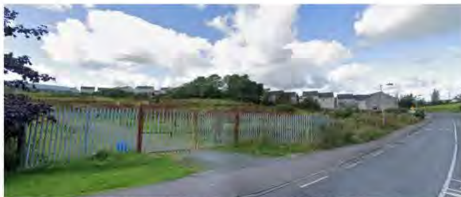
Photo of site prior to works ~ Early 2020
