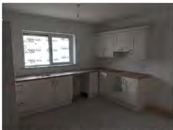
Photo of Kitchen pre flooring ~ October 2020
