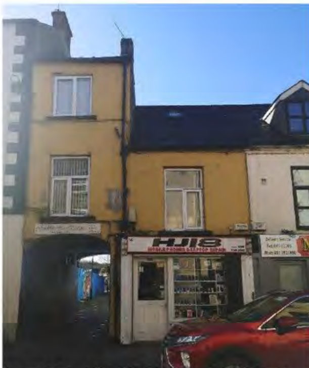
Figure 19: No. 14 Dublin Street – archway through to backlands, Consarc Design Group.
