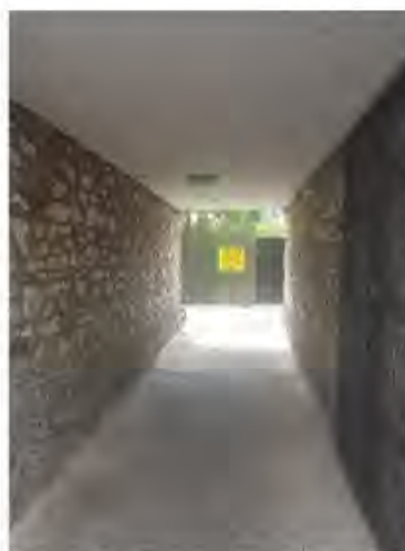
Figure 48: View of alleyway, taken from Dublin Street.
