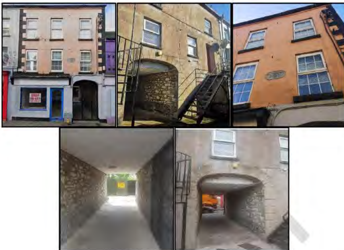
Figure 2: Images of subject building
