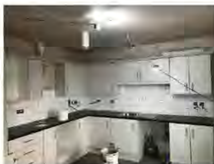
Ready for Snagging for Substantial Completion
