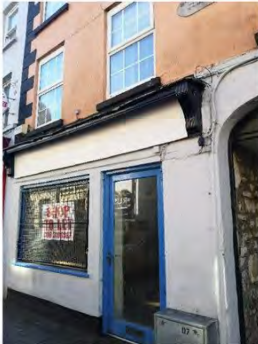
Figure 33: Protected Structures Dublin Street. No. 10 – Shop unit at ground floor level.
