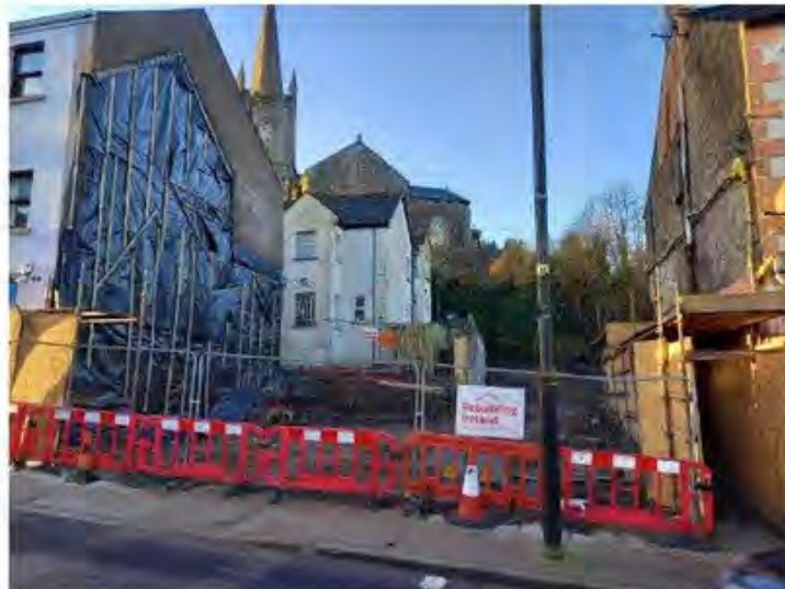
Site 5 "2a & 3 Analore Street" Superstructure Blockwork commenced
