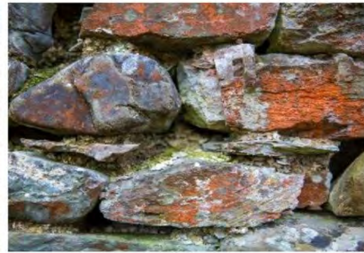
The traditional lime-based mortar used on the wall
