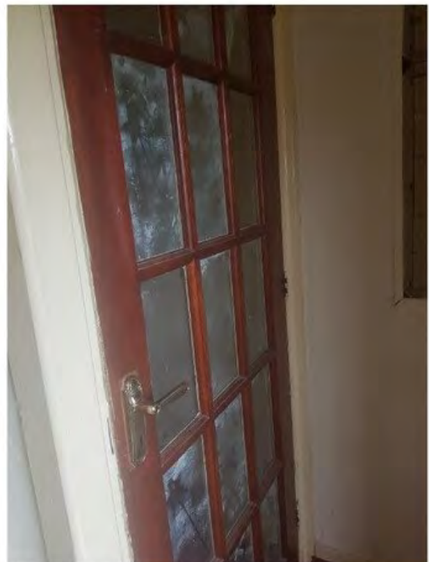
Figure 39: Door to 3rd Floor apartment (no access).
