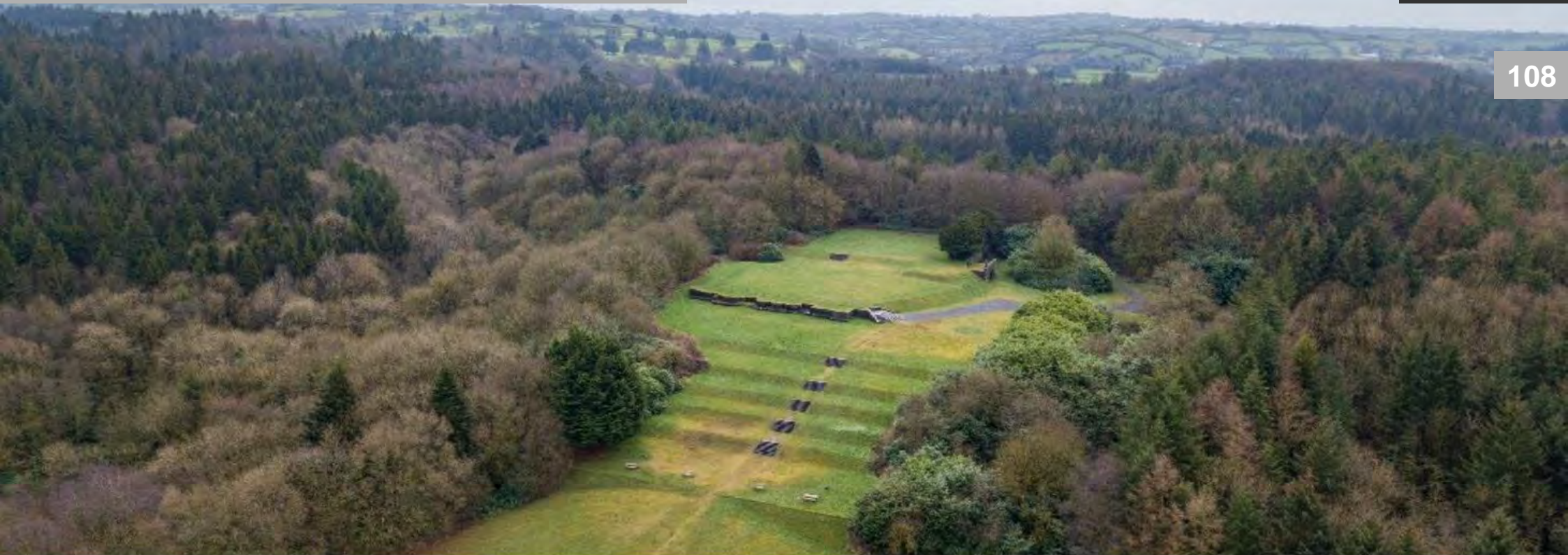
Above: aerial view of the site of Rossmore Castle
