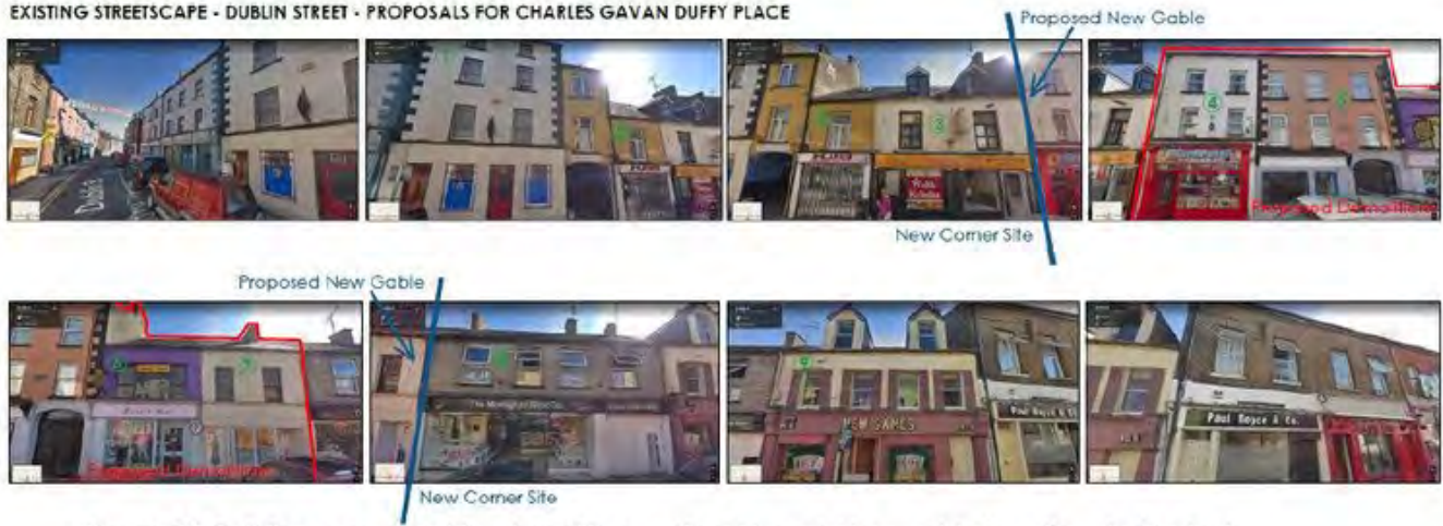
Figure 27: Buildings proposed for demolition outlined in red. New gable locations indicated. Extracts from Google Streetview annotated by Consarc Design Group.
