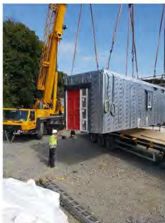
Photo of module being lifted into place ~ September 2020
