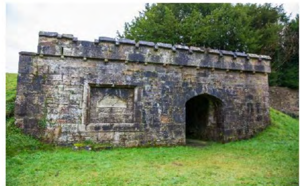
The feature known as the 'Ice House' below the site of Rossmore Castle, likely to be the servants/supplies tunnel
