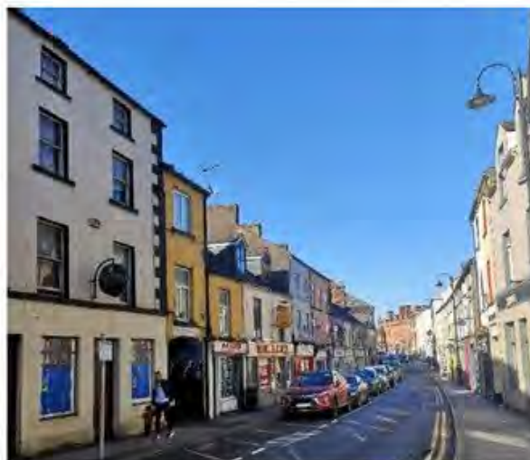
Figure 14: Dublin Street – looking north west. Consarc Design Group
