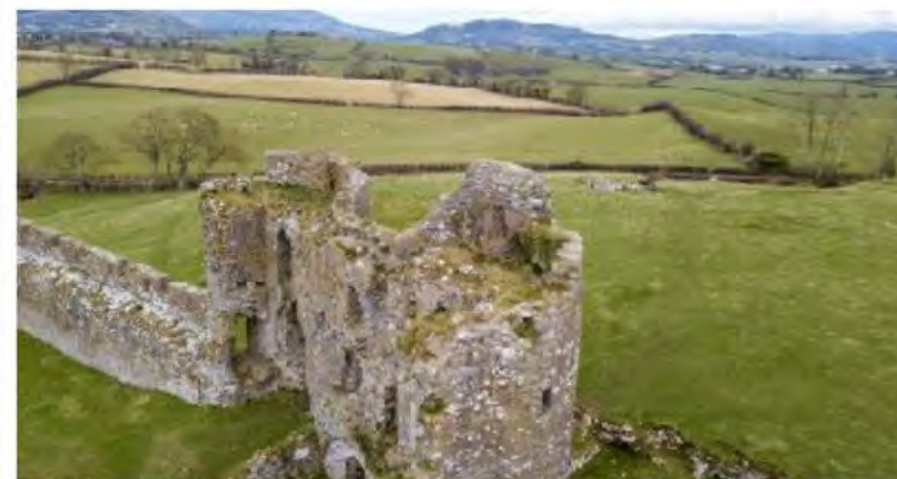
Saplings growing at the top of the towers
