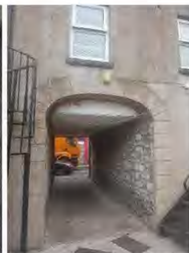
Figure 49: View of alleyway, from rear yard and stair to first floor accommodation.
