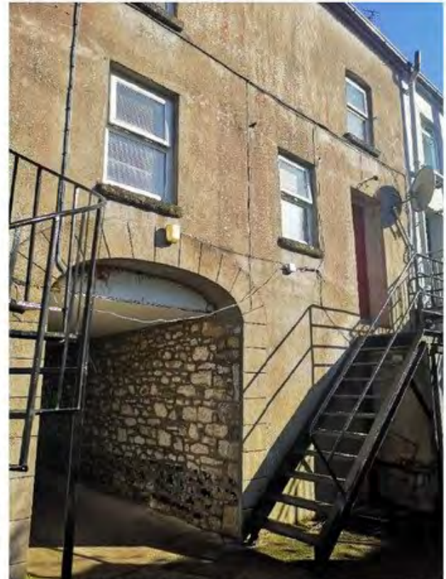
Figure 18: Rear of No. 10 Dublin Street. Consarc Design Group.
