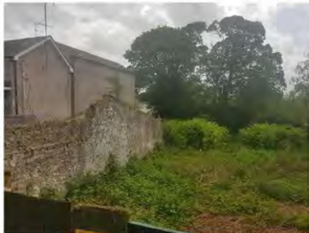
Figure 31: Yard area to rear, gated - photo taken from fire escape stairs.
