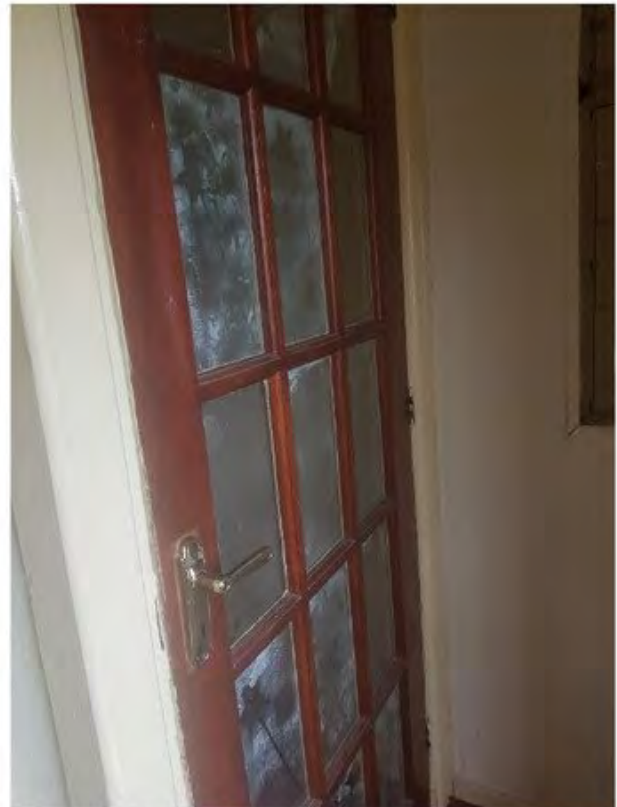
Figure 39: Door to 3rd Floor apartment (no access).
