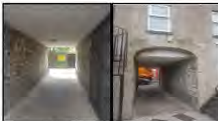
Figure 2: Images of subject building
