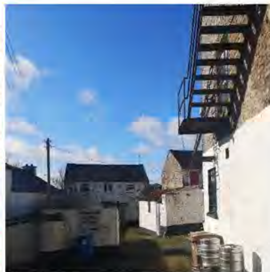
Figure 22: Rear of Sherrys Bar. Consarc Design Group.
