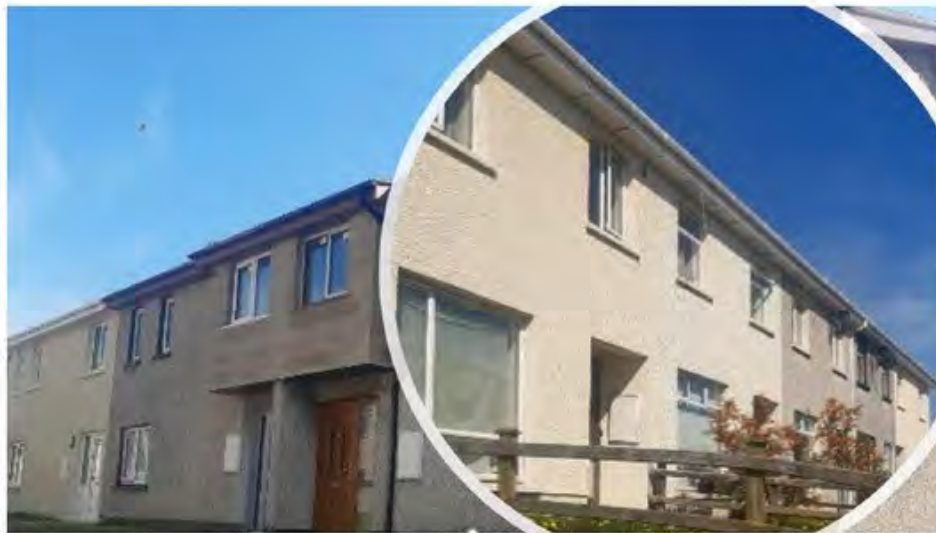
All roof works and bay window works have been completed
