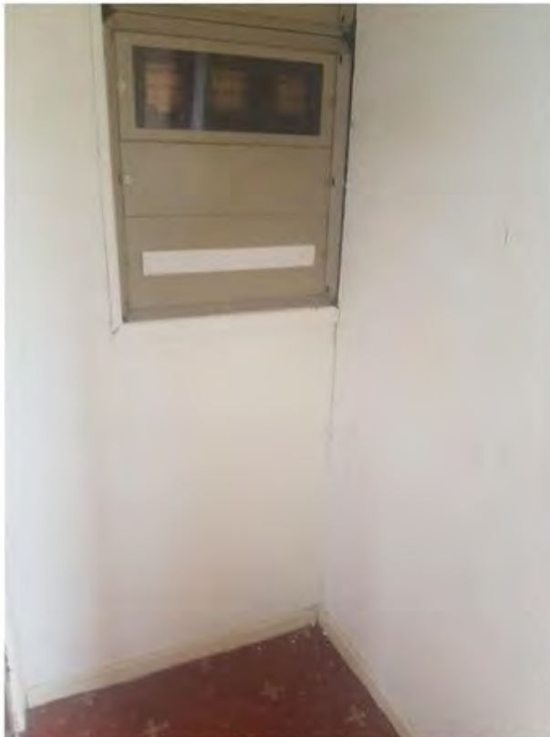
Figure 38: Hallway adjacent to entrance to 2nd floor apartment.
