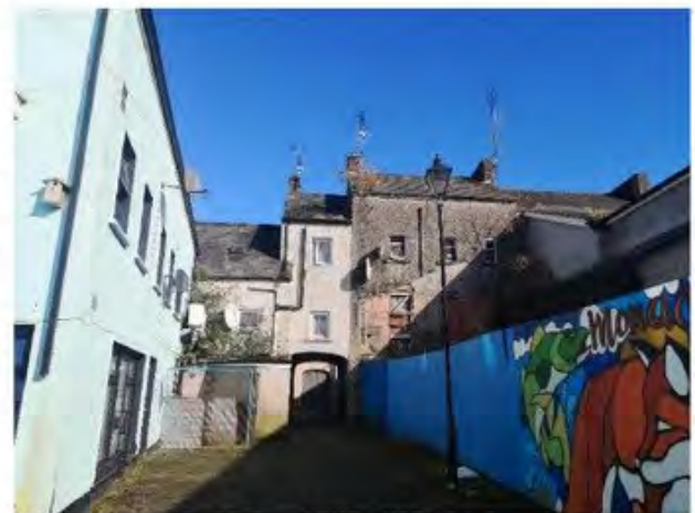
Figure 20: Rear of No. 14 Dublin Street. Consarc Design Group.
