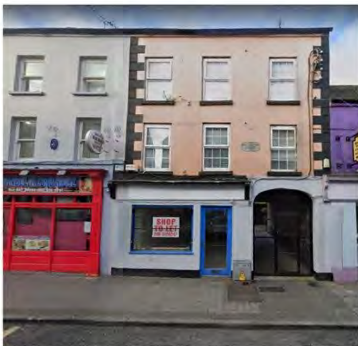
Figure 32: Protected Structures Dublin Street – No. 10 Birthplace of Charles Gavan Duffy. Extract from Google Streetview.
