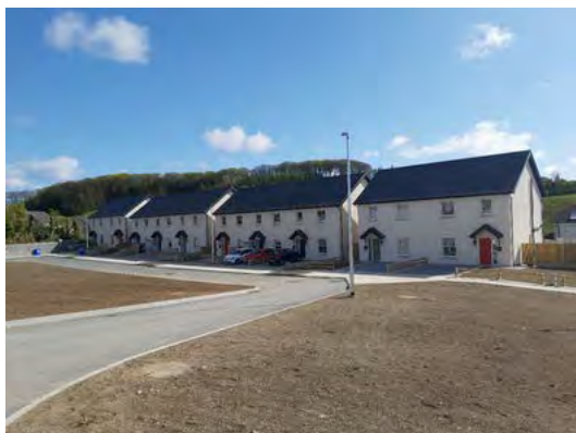
Photo of site works completed: April 2021
