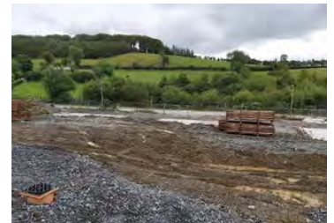
Photo of foundations completed prior to modules arrival: August 2020
