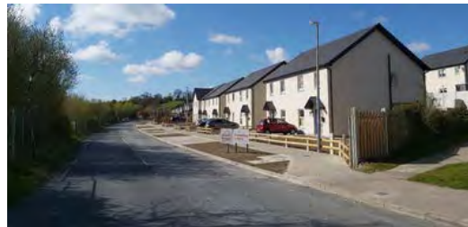
Photo of site works completed: April 2021
