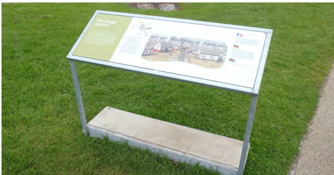
Figure 7.13 The interpretive panels in Vindolanda, Hadrian's Wall, UK, are fitted onto concrete trays. This means that no excavation is required.
