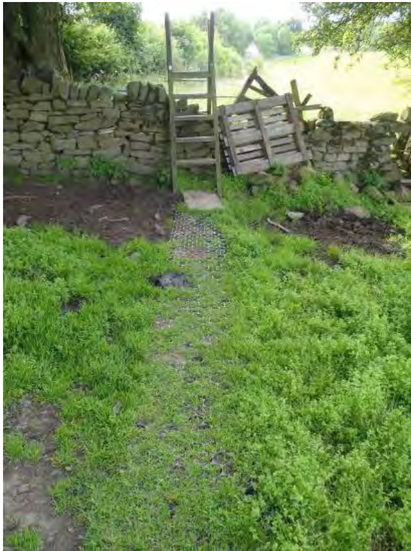
Figure 7.5 Simple plastic mesh along Hadrian's Wall route
