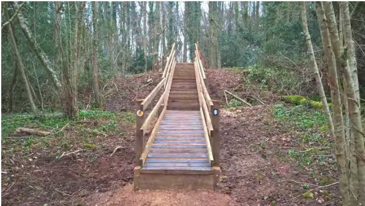
Figure 7.6 Timber boardwalk over Offa's Dyke
