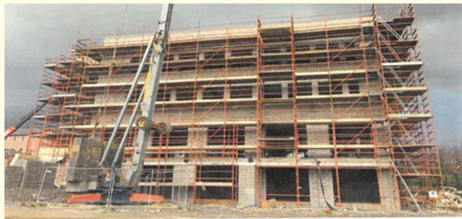
"The Ridge" Enterprise Hub, McGrath Road, Castleblayney
