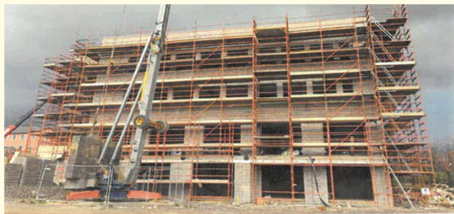
"The Ridge" Enterprise Hub, McGrath Road, Castleblayney
