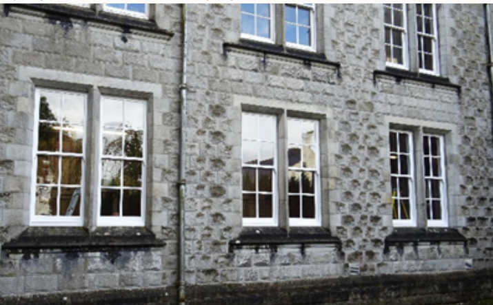
Fig. 2: Window repairs to Teach Iosef, St. Louis Secondary School, Monaghan
