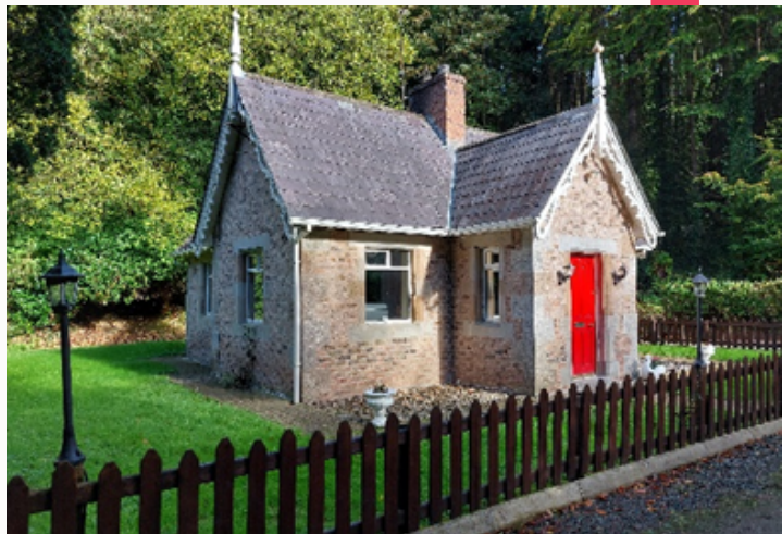
Fig 1: Repair of the finials at Newbliss Gate Lodge, Rossmore
