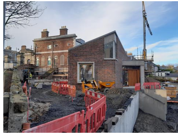
Ongoing Library Construction
