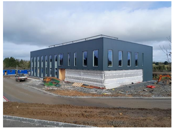
Ongoing Bioconnect Construction
