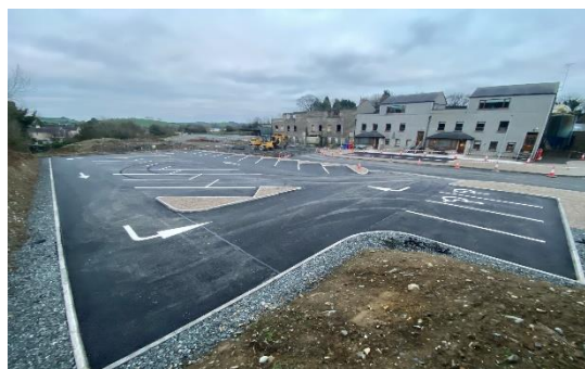
Ballybay courtyard carpark
