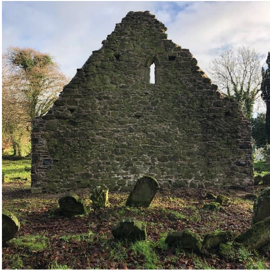
Killeevan Wee Abbey after conservation works to the gable were completed.
