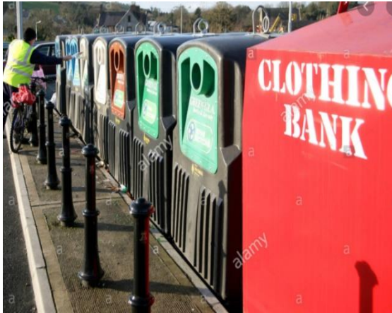
Bring facility at Drummond Etra, Carrickmacross
