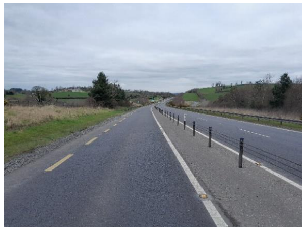
N2 Tullyvin to Lislanly Pavement Rehabilitation scheme
