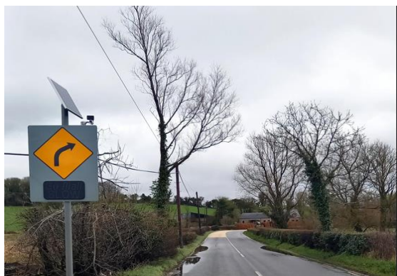
R183 Low Cost Safety Improvement Works after
