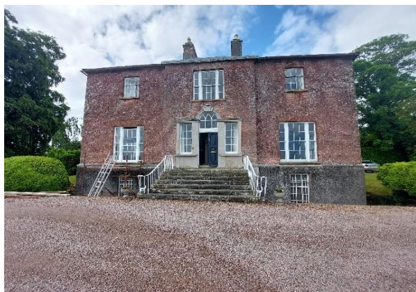
Conservation repairs to windows at Freame Mount House, Dartrey
