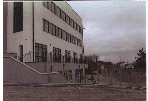
"The Ridge" Enterprise Hub, McGrath Road, Castleblayney
