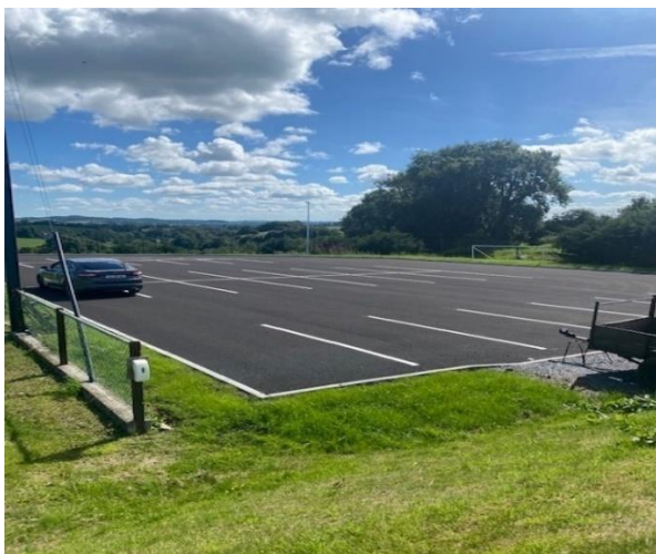
Clones Town FC Car park facilities
