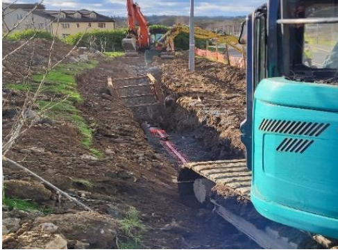
Construction Work Carrickmacross WWTP
