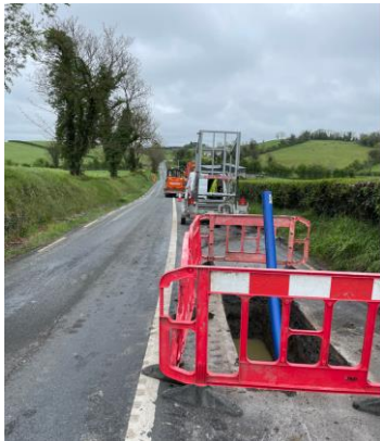
Water Mains replacement Newbliss (2)
