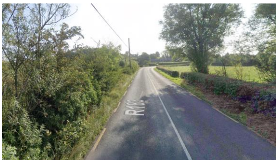
R183 Low Cost Safety Improvement Works before
