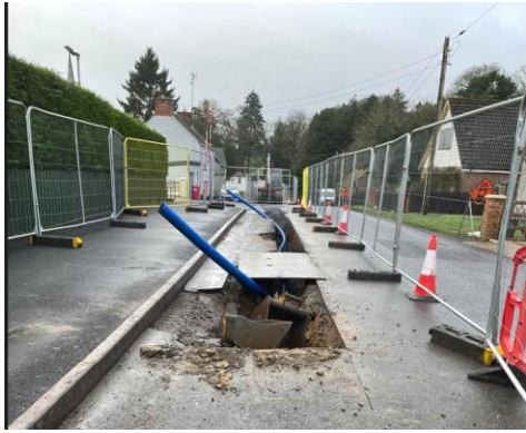
Water Mains replacement Newbliss (1)
