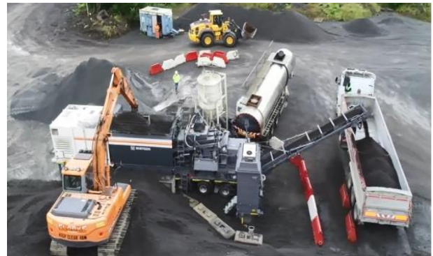
Reclaimed Asphalt Quarry Processing in Glenmore Quarry, Carrickroe
