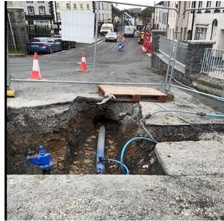
Water Mains replacement Castleblayney
