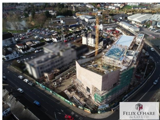
MPC- Works Progressing East Face
