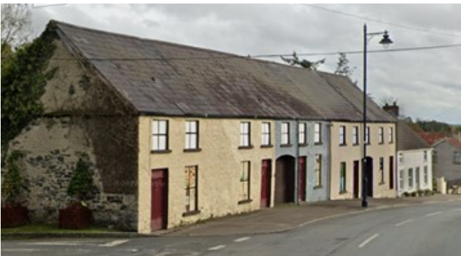
Evelyn Terrace and Semi Detached Residential Structures—Long Term Vacant properties in the village centre Vacant Homes
