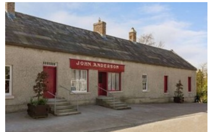
Drum: Andersons Vernacular Refurbished Protected Structure
