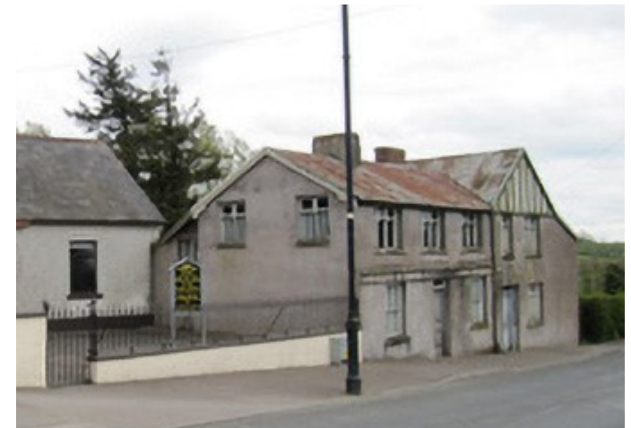
Drum—Vacant Dwellings adjoining the Gospel Hall
