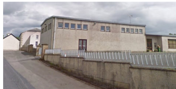
Hall adjoining Drumcorrin National School
