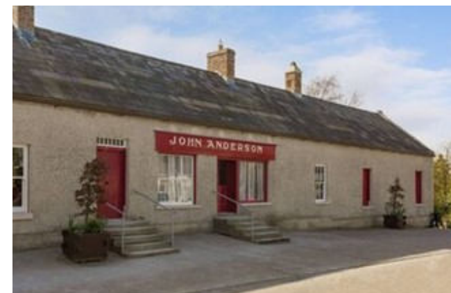
Drum: Andersons Vernacular Refurbished Protected Structure
