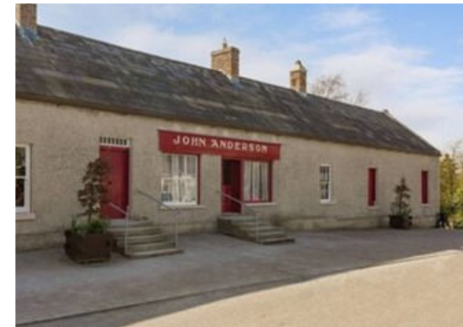
Drum—John Anderson house and shop
