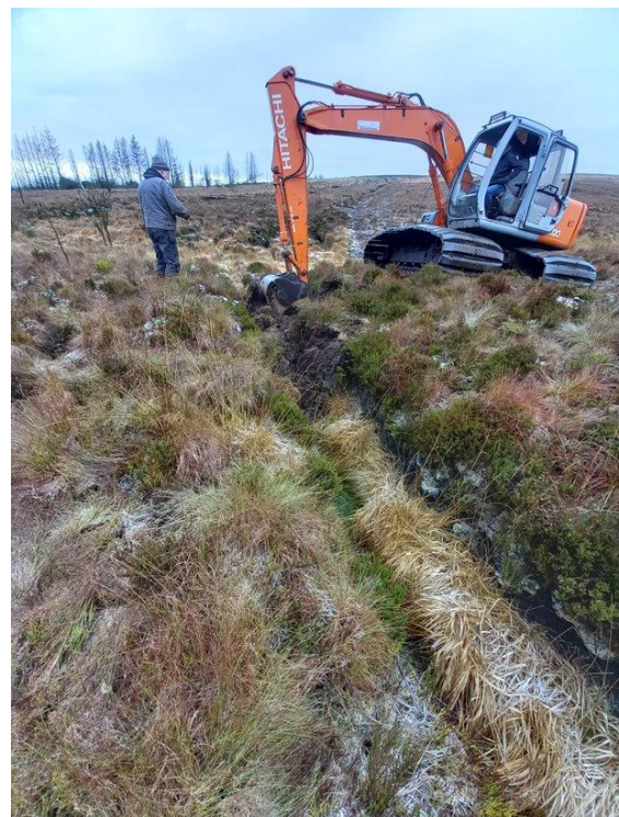
Creating a peat dam to block drain on Sliabh Beagh to restore the hydrological functions of the blanket bog.
