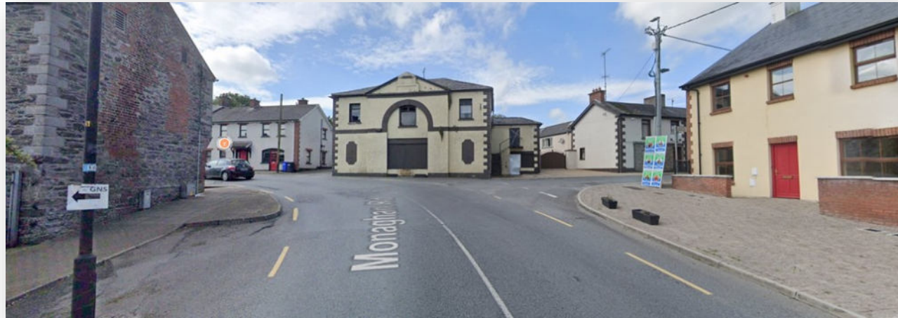
Existing Street View – Poorly presented streetscape / vacancy, expansive roadway and vehicular priority
