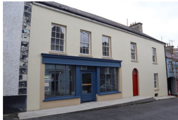
Ramelton Co Donegal —Adaptation and Reuse of historic dwelling, reinstatement of shopfronts, and reinstatement of lime render by Dedalus Architects Illustration of before and after
