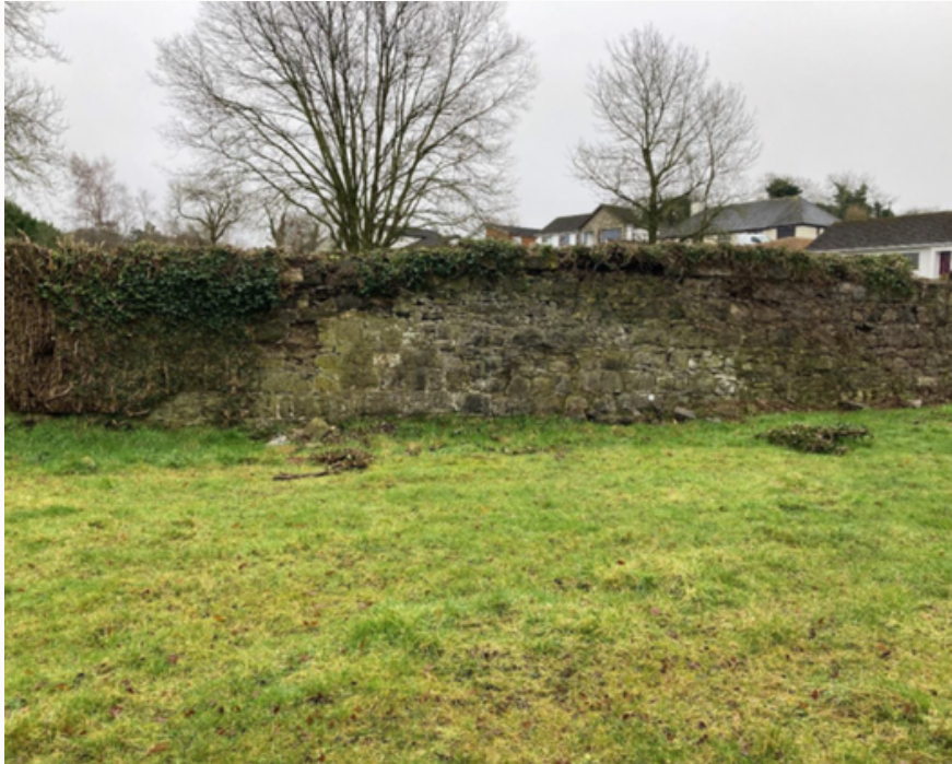
Wall at Glaslough Railway Station before works
