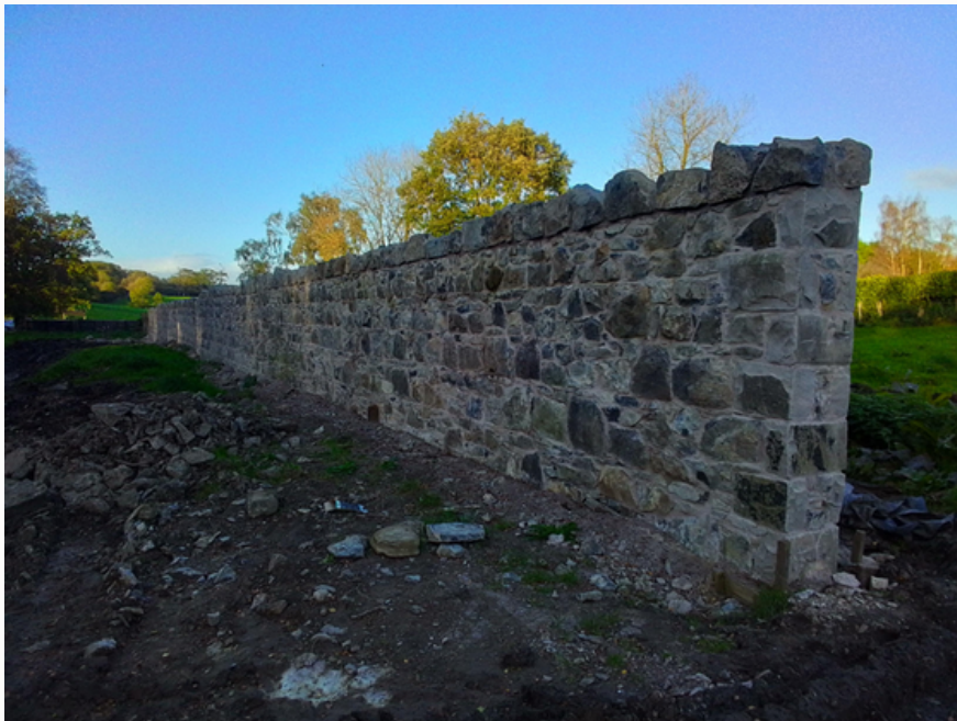
Wall at Glaslough Railway Station after works completed
