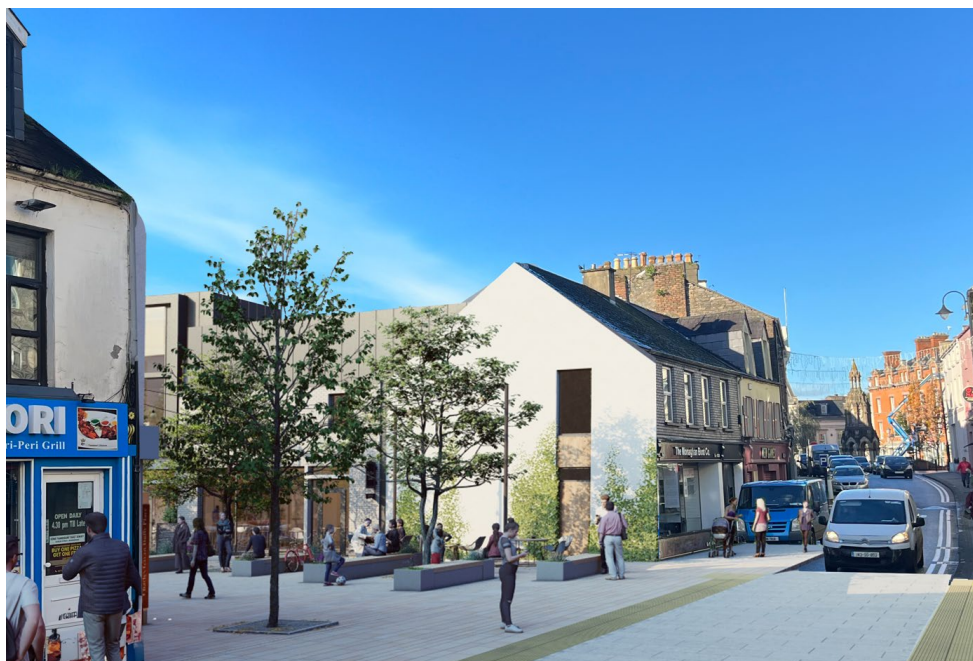
Figure 2.15: Photomontage showing the proposed elevation on the new gable of No 7 Dublin Street (Monaghan Boot Co)
