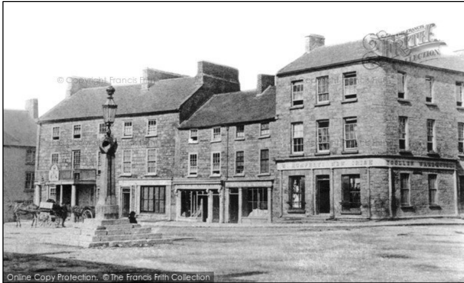
Figure 15.9.6.2: The Diamond c.1870 (Francis Frith Collection) – Alma House on the corner of Glaslough Street and market cross to the centre.
