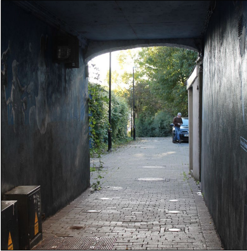
Figure 15.9.7.5.4: Existing access route through archway to carparking area proposed for new development site.
