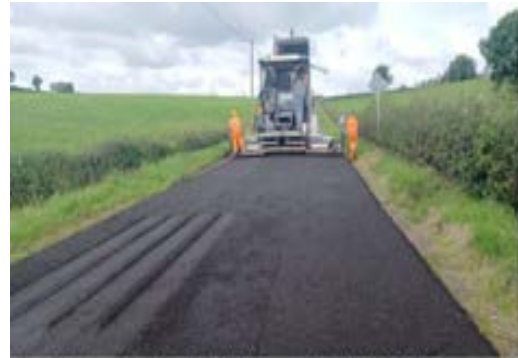
Figure 1 : Laying of Reclaimed Asphalt Pavement on the LP1210 at Derrygasson Lower
