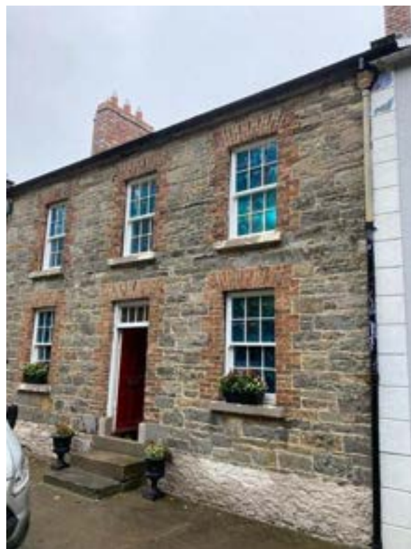
Conservation repairs to windows & roof at 25 Main Street, Glaslough
