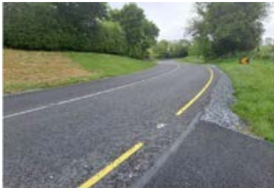
Figure 3: Restoration Improvement Grant. Surface Overlay strengthening works of the R 142 at Killyvine
