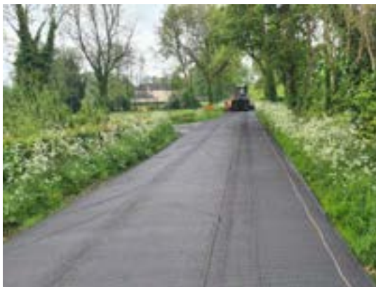
Figure 3: Restoration Improvement Grant. Surface Overlay strengthening works of the R 142 at Killyvine
