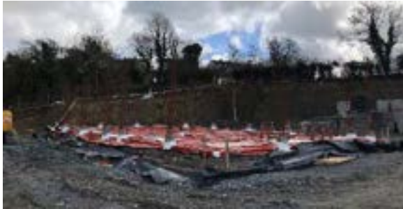
Construction of new Ballybay Fire Station
