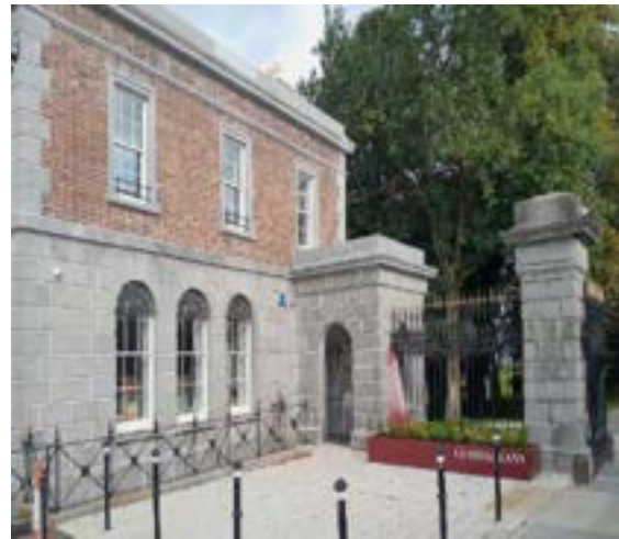
Refurbished Gate Lodge Library Building
