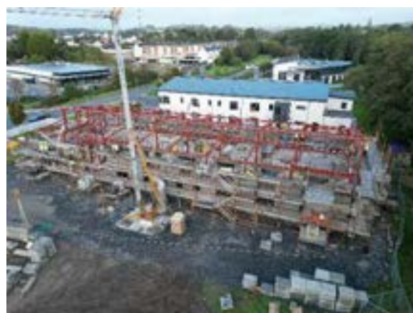
C:TEK II Co-working Enterprise Hub under construction
