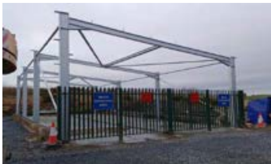
Works at new storage compound – Feb 2024
