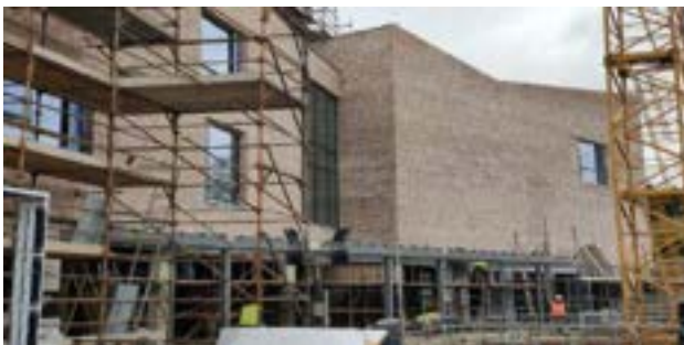
The exterior of the museum-end of the building
