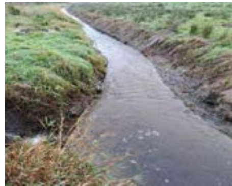
Kilmore East, flood alleviation works
