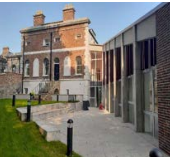
Refurbished Gate Lodge Library Building
