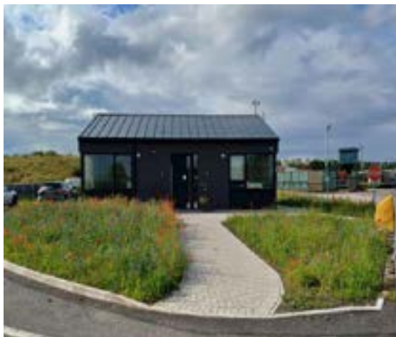
New Landfill Site Office Building
