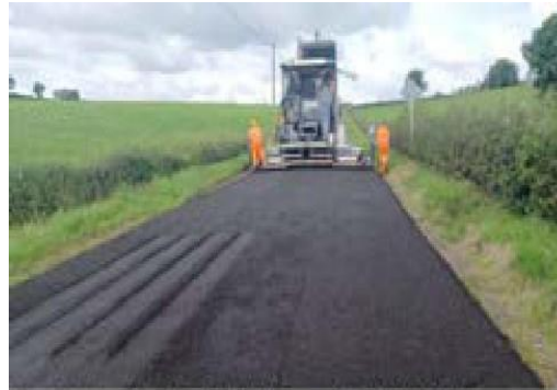
Figure 11: Laying of Reclaimed Asphalt Pavement on the LP3230 at Derrygasson Lower
