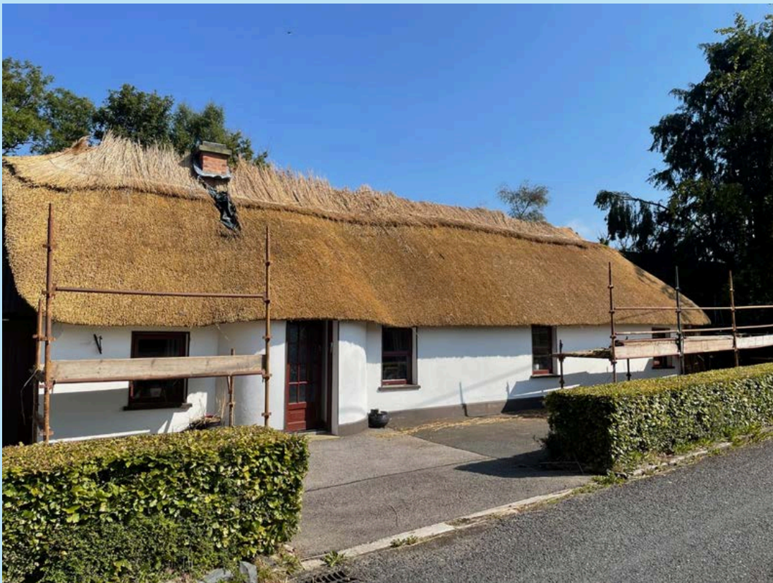
Thatching work reaching completion at Greenan's Cottage
