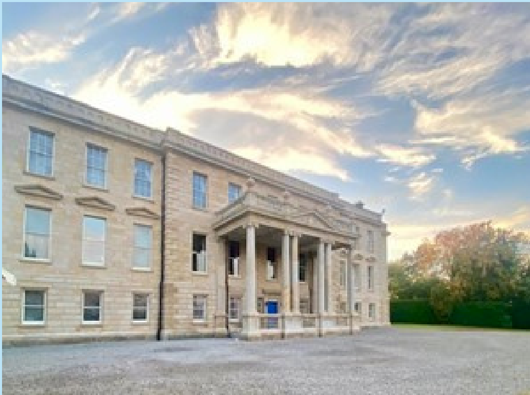
Hilton Park after stonework restoration.
