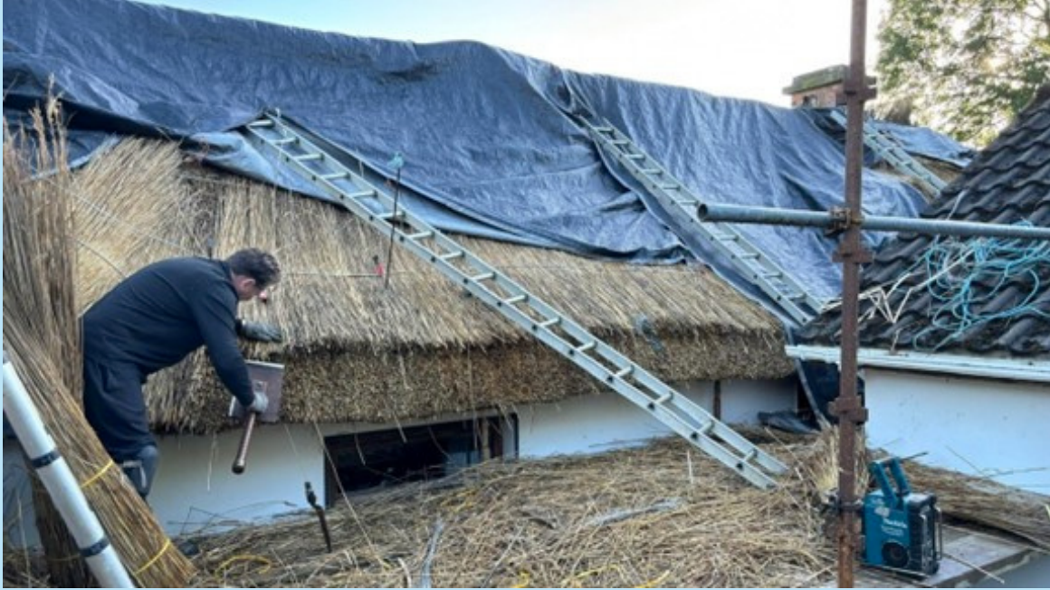
Thatching work ongoing at Greenan's Cottage
