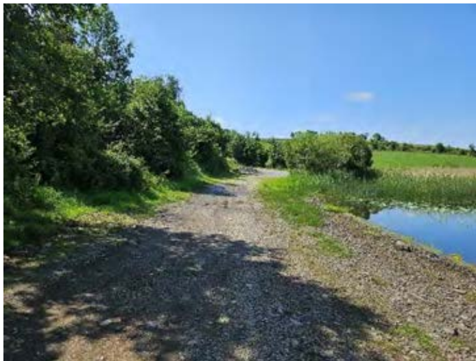
Existing Road Conditions
