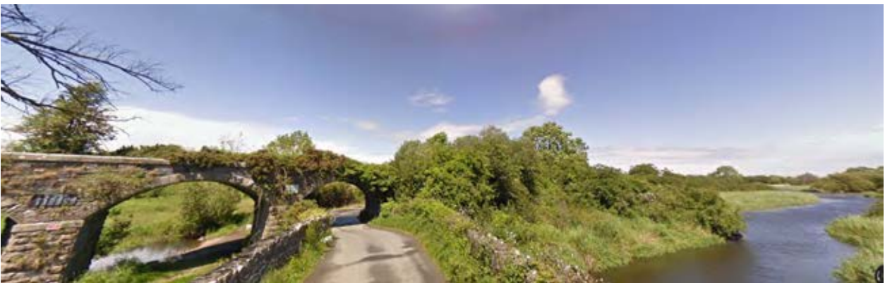
Photo taken from Google Street View is taken from the Ballymascarra Bridge looking north and shows the road passing under the railway embankment with the bridge over the river shown to the left.
