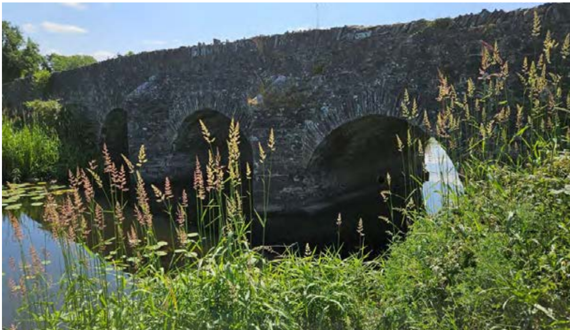
Bridge as viewed from river foreshore.
