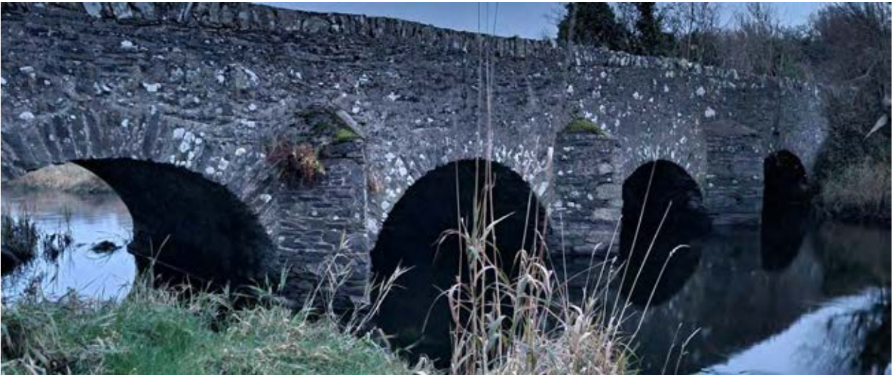
Photo shows the Ballymascarra Bridge looking at it from the downstream side. The subject site is located to the right of the bridge. It is thought that in times of flood that this bridge acts as somewhat of a throttle for the flow causing water to cross the road to the south of it.
