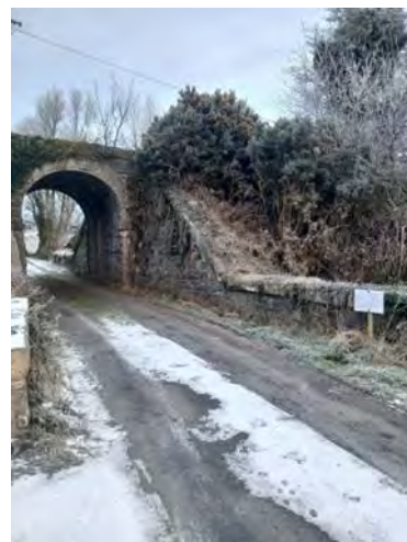
Site Notice at Ballynascarva Bridge (Lisnalong)
