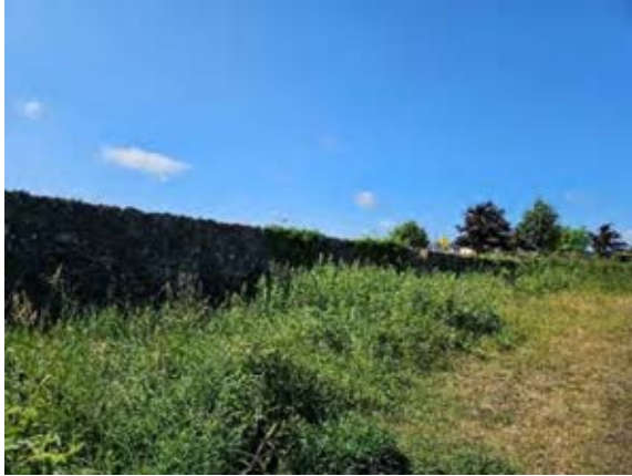
Bridge is a protected structure , ref no, 414023.
