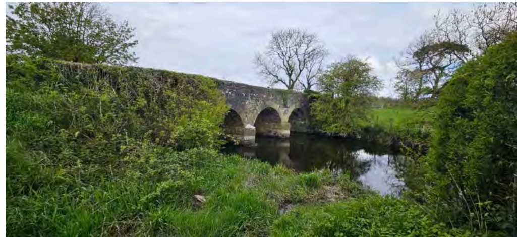
Plate 8: Balladian Bridge with existing slipway in foreground
