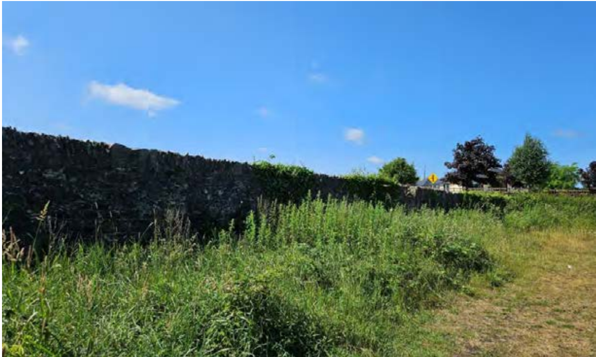
Wing wall to bridge to the east of the bridge adjacent to the proposed hardstanding.
