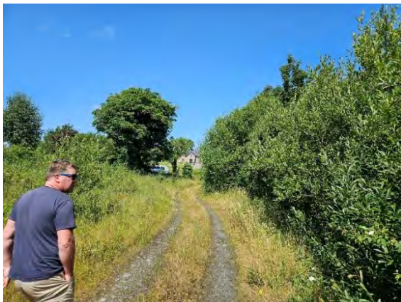
Existing Internal Road
