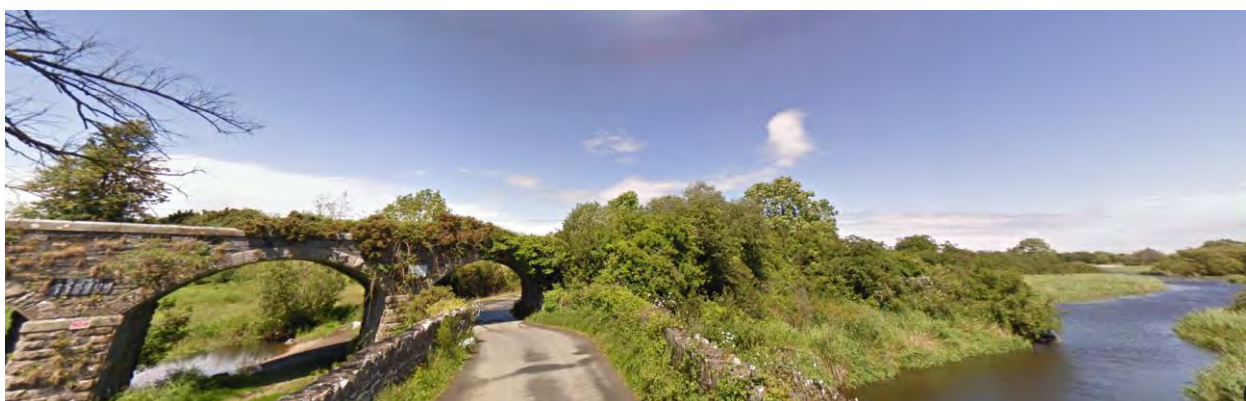
Photo taken from Google Street View is taken from the Ballymascarra Bridge looking north and shows the road passing under the railway embankment with the bridge over the river shown to the left.
