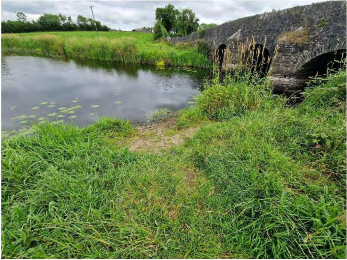
Plate 7. Photo of proposed works location at Ballycoghill Bridge
