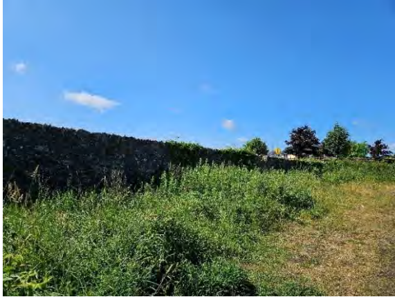
Bridge is a protected structure , ref no, 414023.
