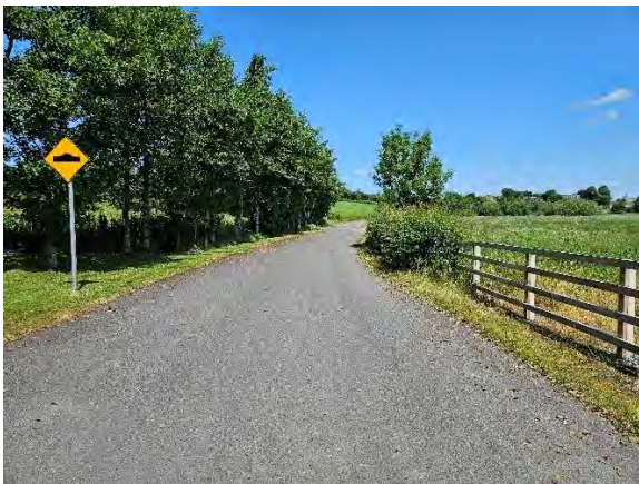
Road in good condition-No roadworks proposed
