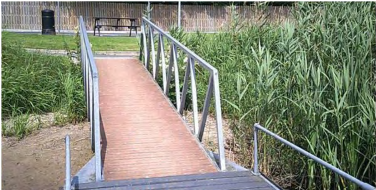
Existing access at Lough Major, Ballybay at Blueway Trailhead
