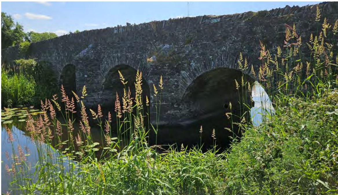
Bridge as viewed from river foreshore.
