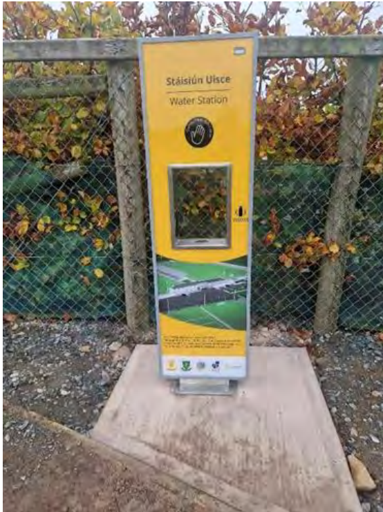
Clontibret O'Neills GAA – installation of water refill station
