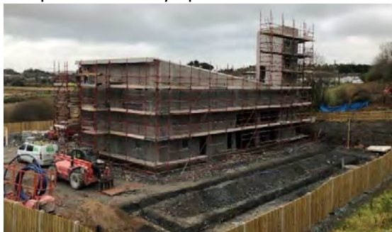
Construction of New Ballybay Fire Station Nov 2024
