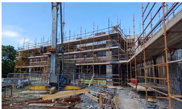
Building Control Inspection Scoil Mhuire National School Rockcorry: July 2024.
