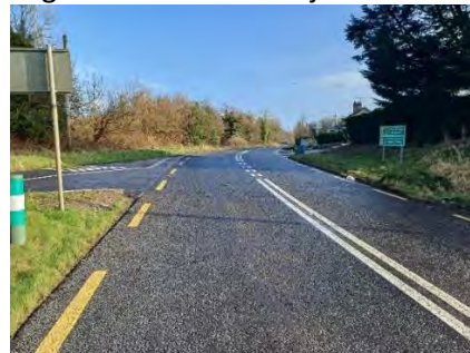
N12 Road Safety Improvement Scheme on N12, Skinnagin.
