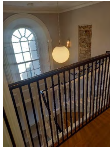
Newbliss- Stairs & Landing
