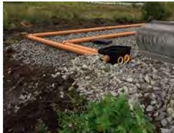
Example of works carried out on a Domestic Wastewater Treatment System
