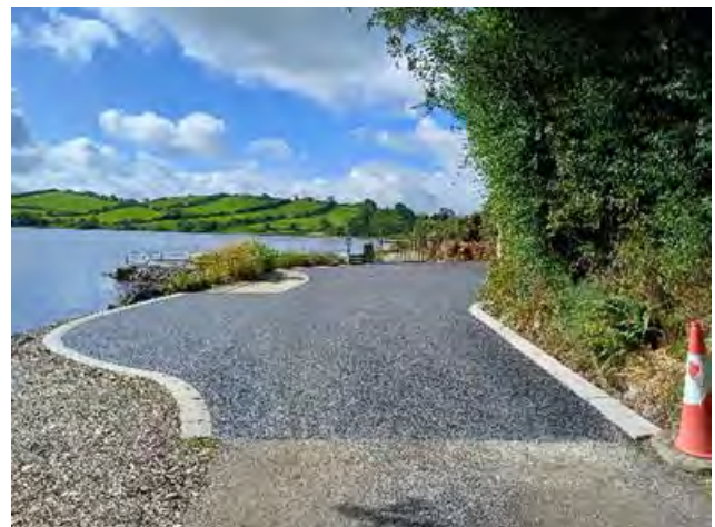
Upgrade of jetty and carparking at Lough Nagarnaman
