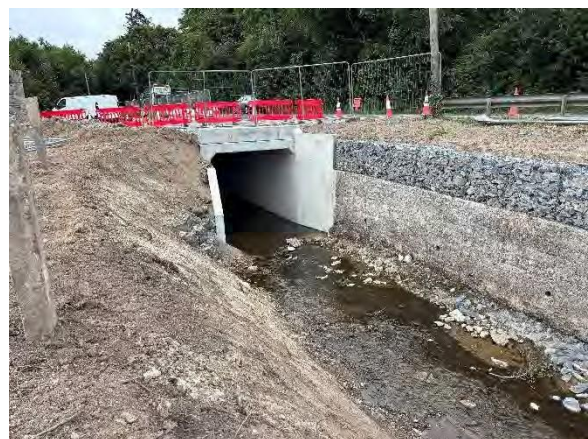
Sheetpiling & Culvert repairs @ Derrylavan
