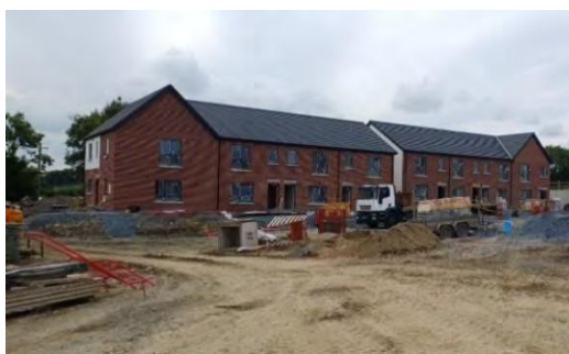
Building Control Inspection: Gleann Dromin July 25
