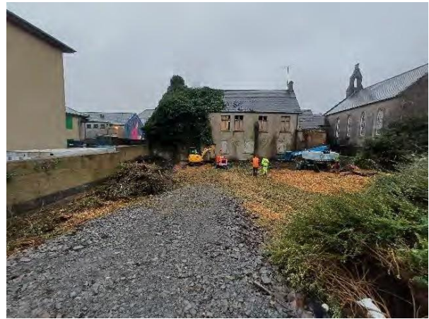
Assembly rooms rear, vegetation being removed
