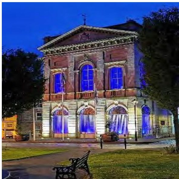
Clones Municipal Offices
