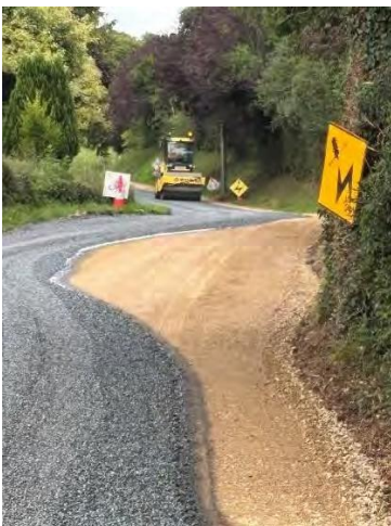
Low-cost intervention works on the LP4510, Donaghmoyne
