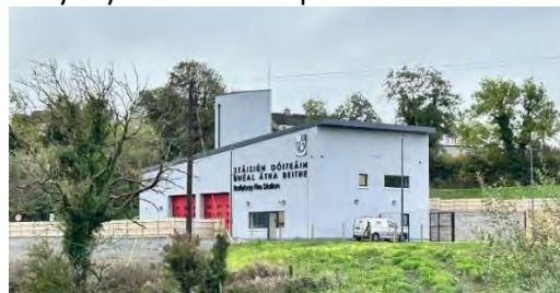
New Ballybay Fire Station Oct 2025
