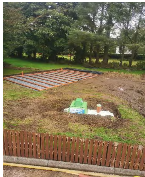
Example of works carried out on a Domestic Wastewater Treatment System
