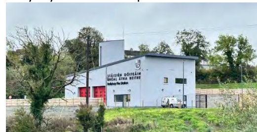
New Ballybay Fire Station Oct 2025
