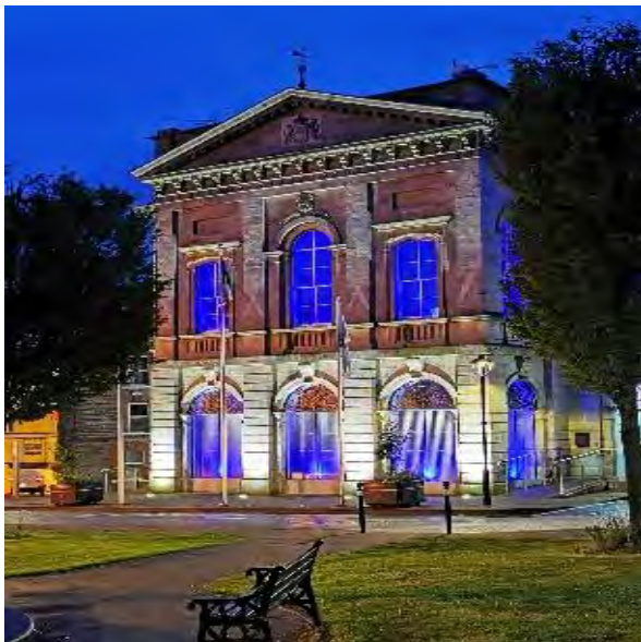
Clones Municipal Offices
