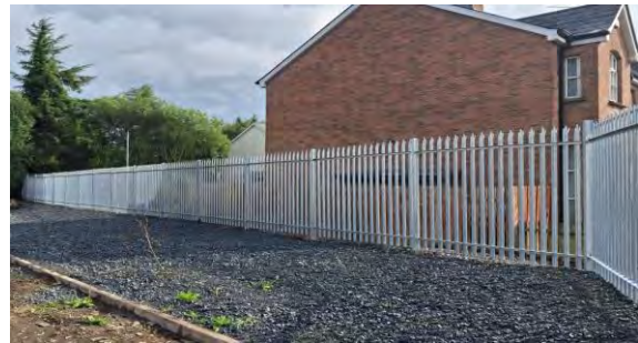
Fencing erected on site in Castleblayney under the ADI Program
