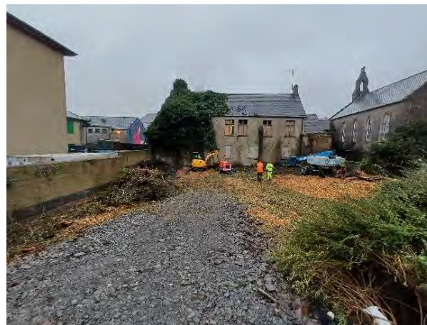
Assembly rooms rear, vegetation being removed
