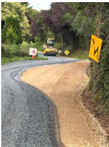
Low-cost intervention works on the LP4510, Donaghmoyné
