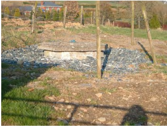
Example of works carried out on a Well
