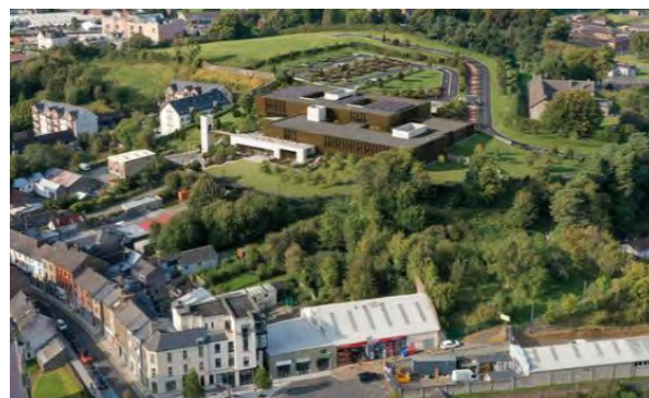
3D Birdseye CGI image of the proposed new Civic Offices at Roosky
