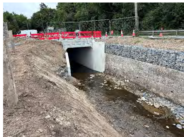
Sheetpiling & Culvert repairs @ Derrylavan
